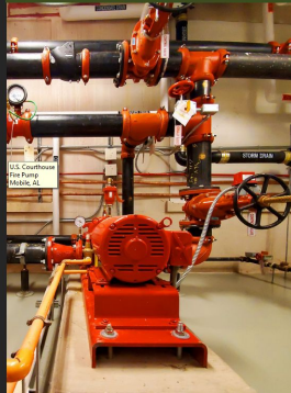
Figure 12. U.S. Courthouse, Mobile, AL
