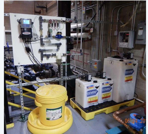
Chemical containers and side stream filtration system used by the chemical scale inhibition system. Photo credit Doug Baughman, GSA
