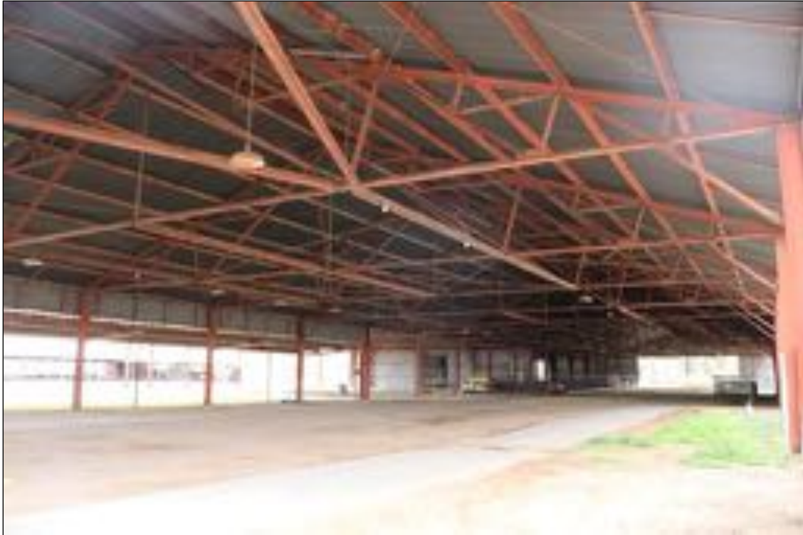
Figure 225. Holding Area Shelter metal frame, looking south.
