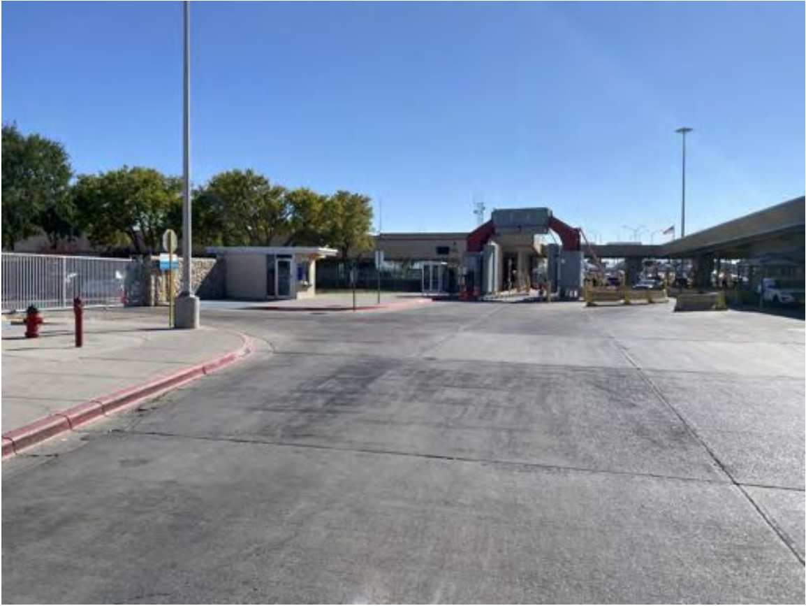
Photograph 1: View looking south of the northern end of the facility.
