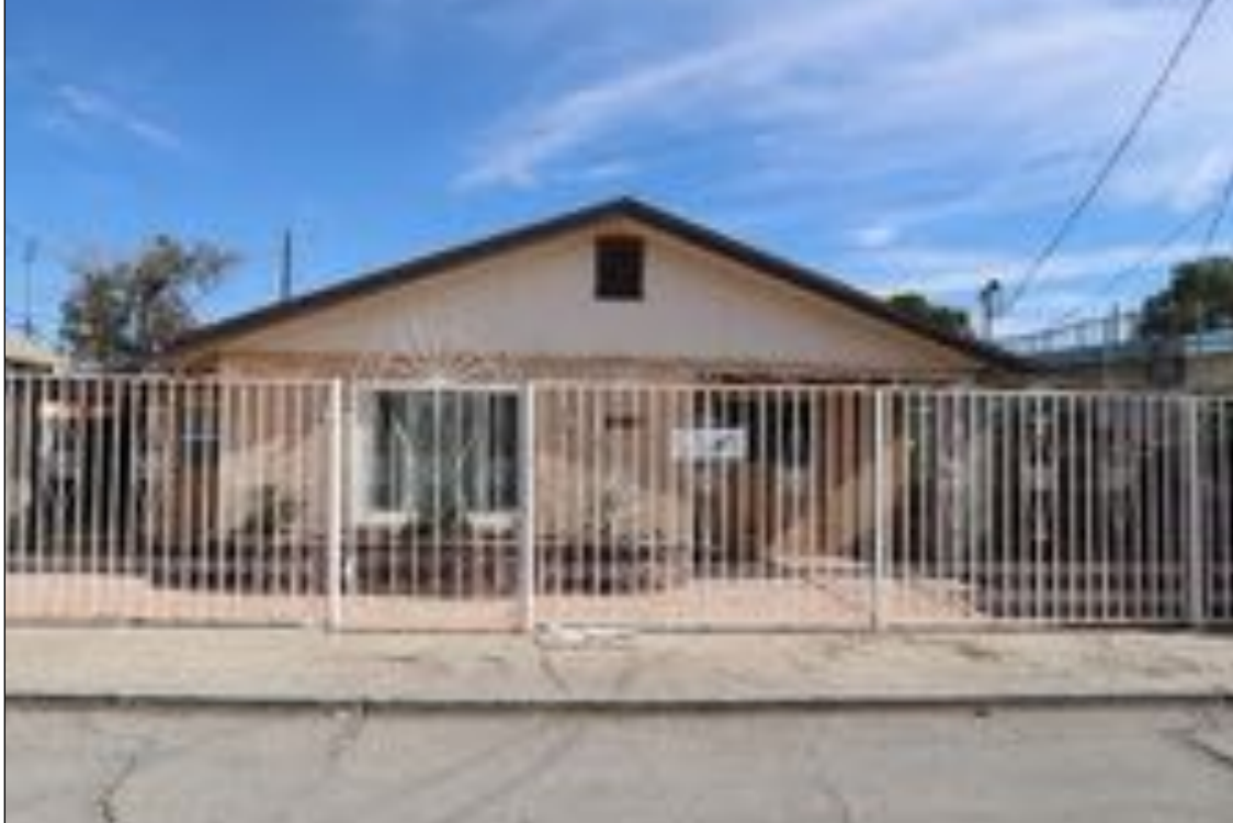
Figure 104. 220 Hardesty Place (Residence), looking east.
