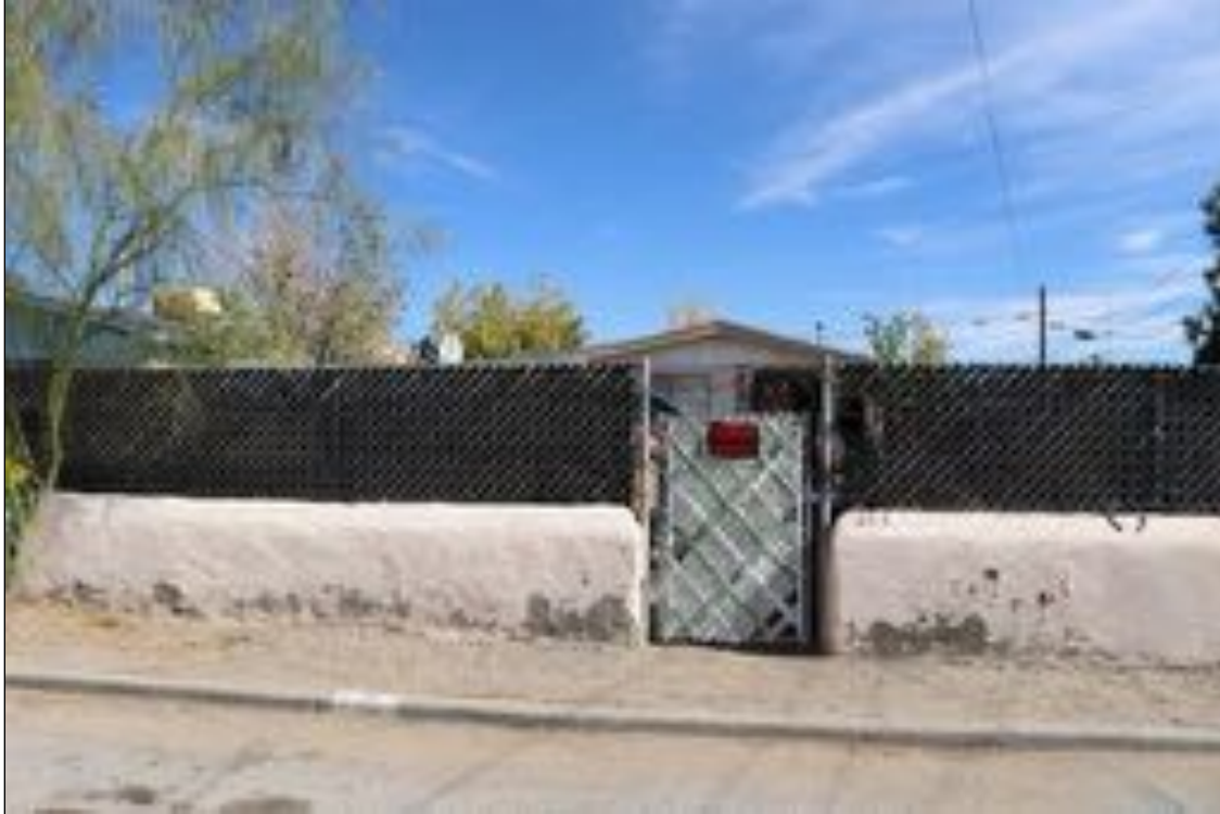
Figure 100. 216 Hardesty Place (Residence), looking east.
