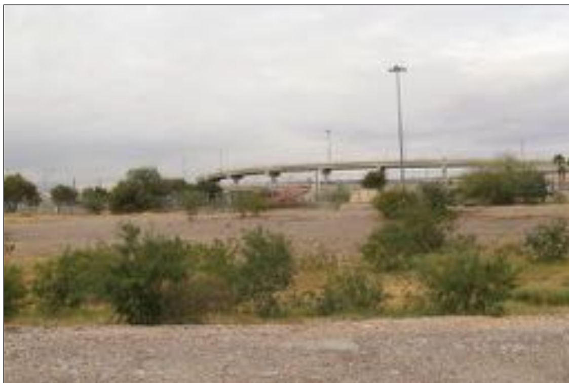
Figure 11. Retention Pond, looking southwest.
