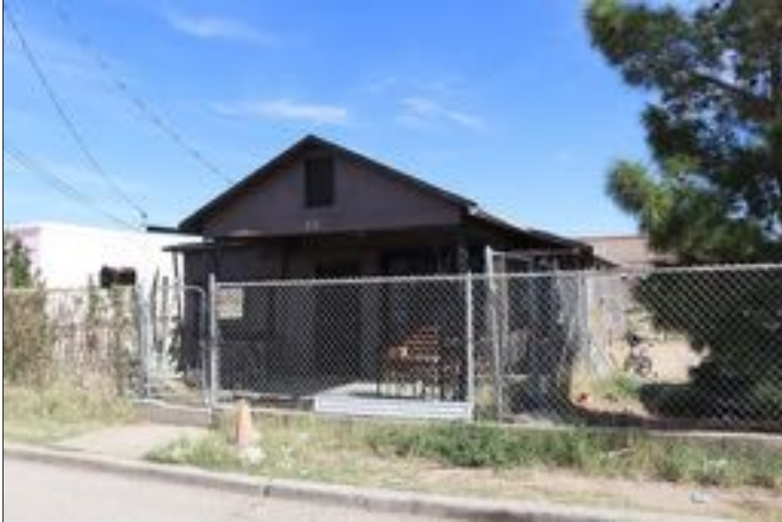
Figure 95. 212 Hardesty Place (Residence), looking northeast.
