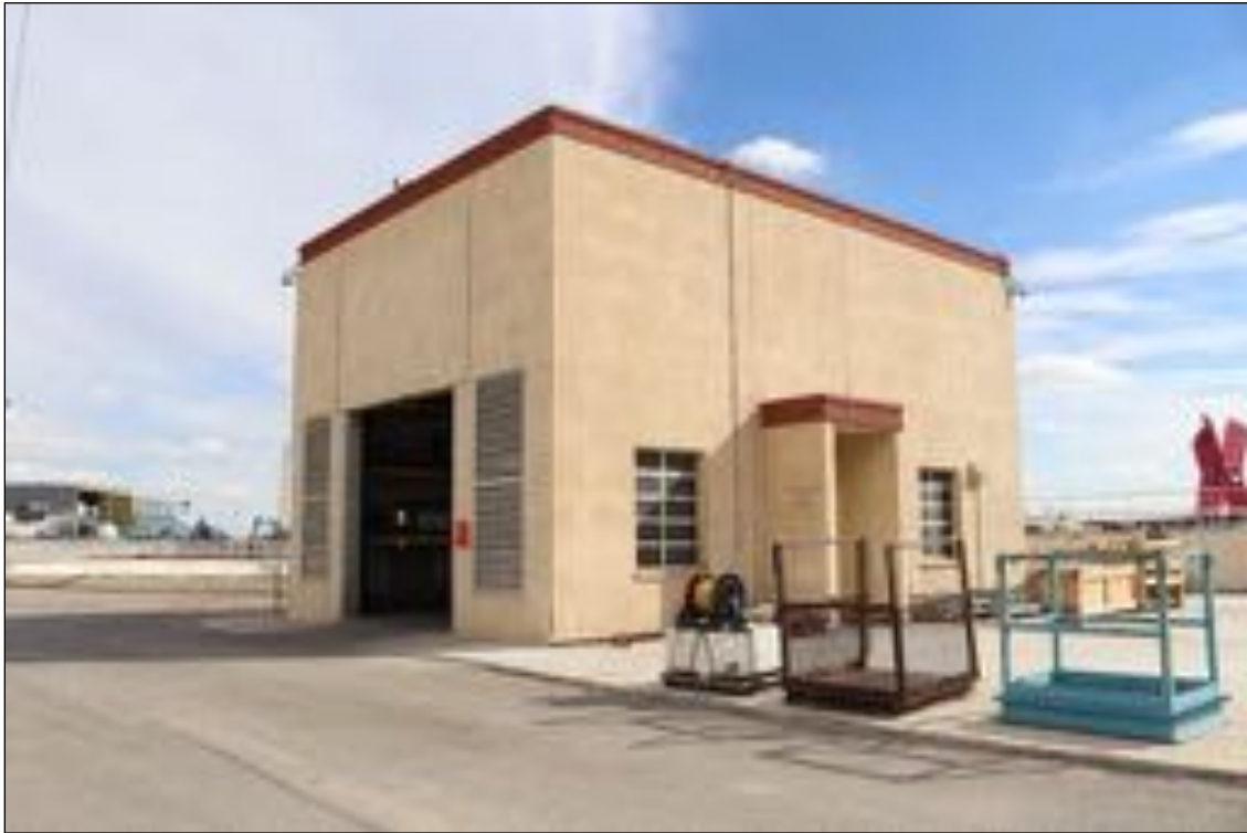
Figure 263. Oxygenation Supply System Building, looking southeast.
