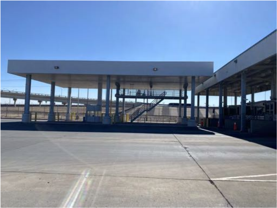
Photograph 7: View looking south of the truck primary inspection area.
