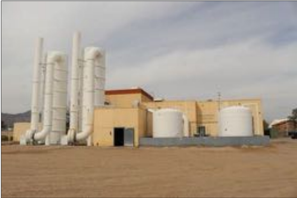
Figure 255. Headworks Building, looking north.
