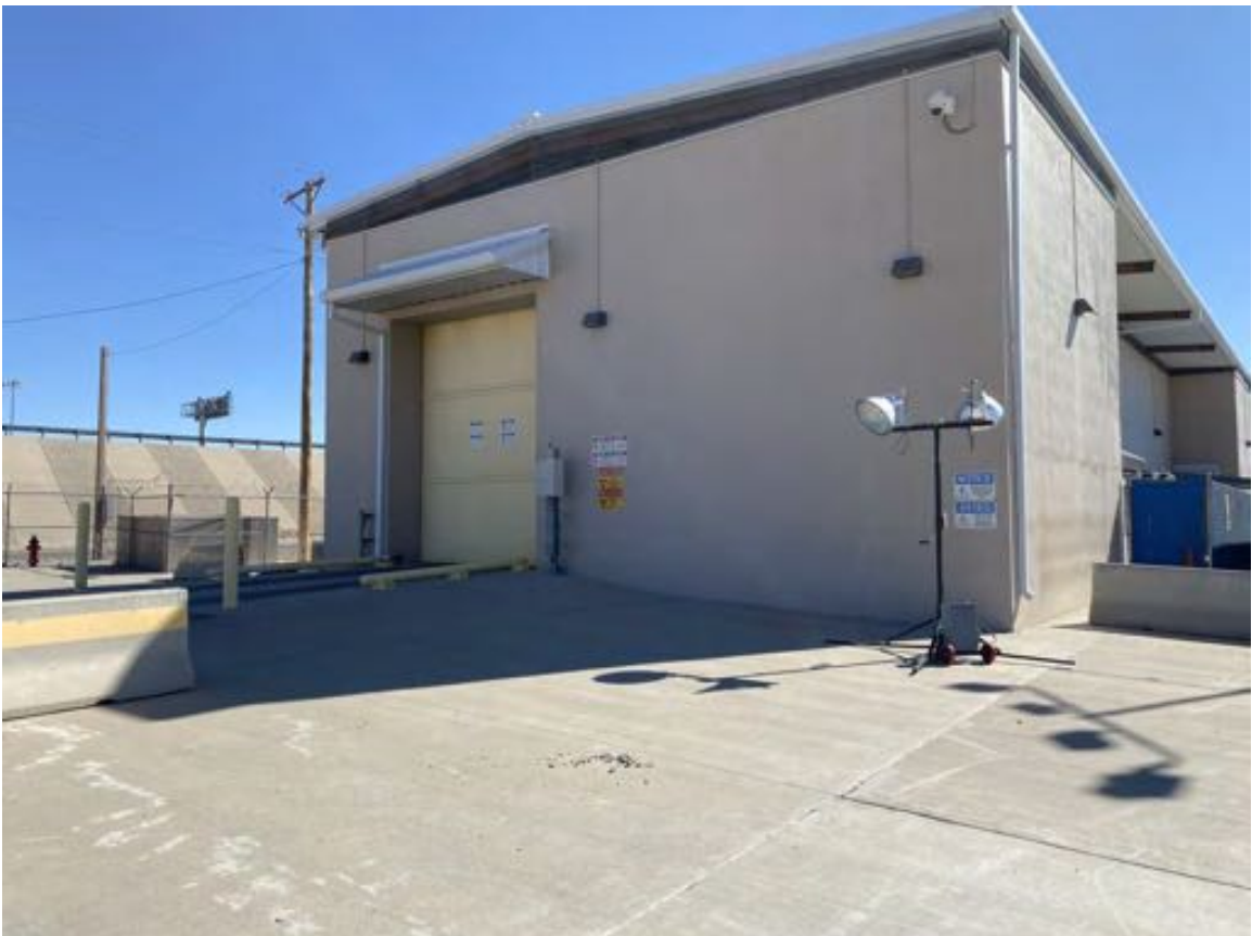
Photograph 8: View looking south of the gantry building.
