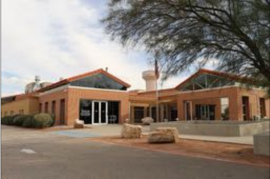
Figure 22. El Paso Water International Water Quality Lab, looking southwest.
