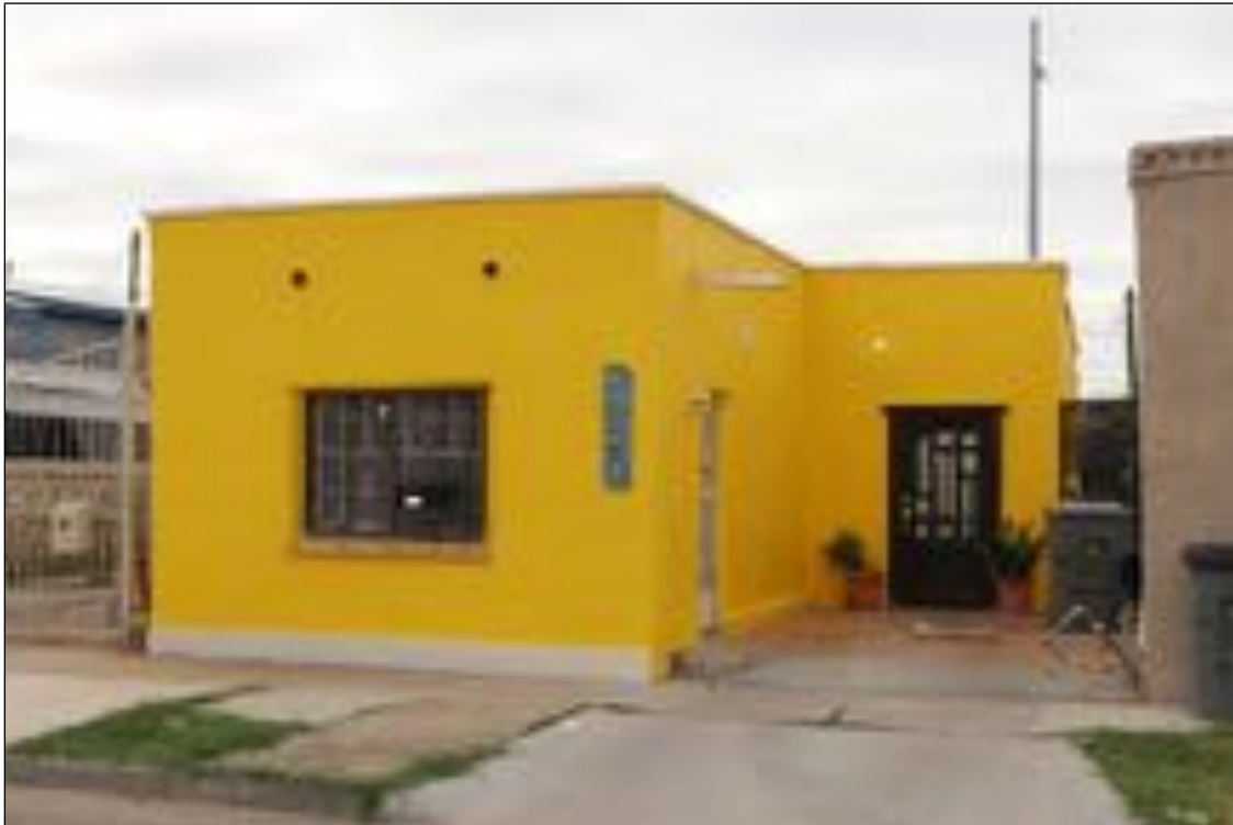
Figure 191. 3820 E San Antonio Avenue (Residence), looking south.
