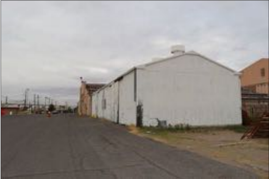
Figure 221. Storage Building, looking west.
