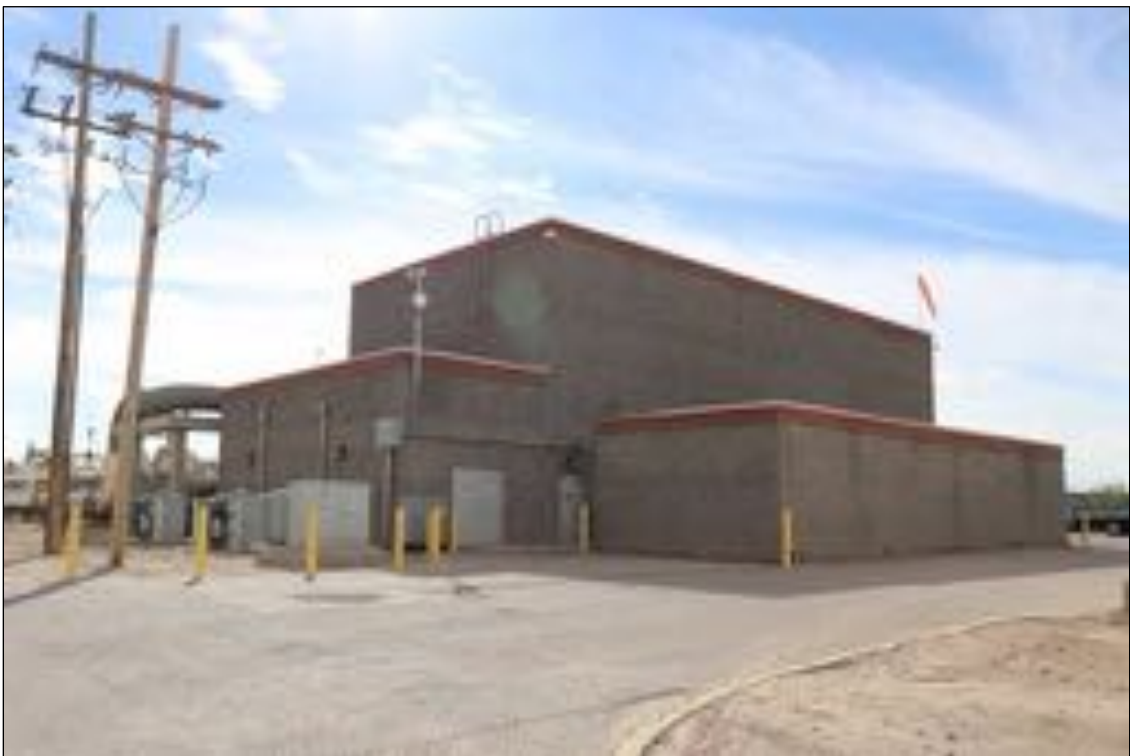
Figure 261. Engineering, looking southwest.
