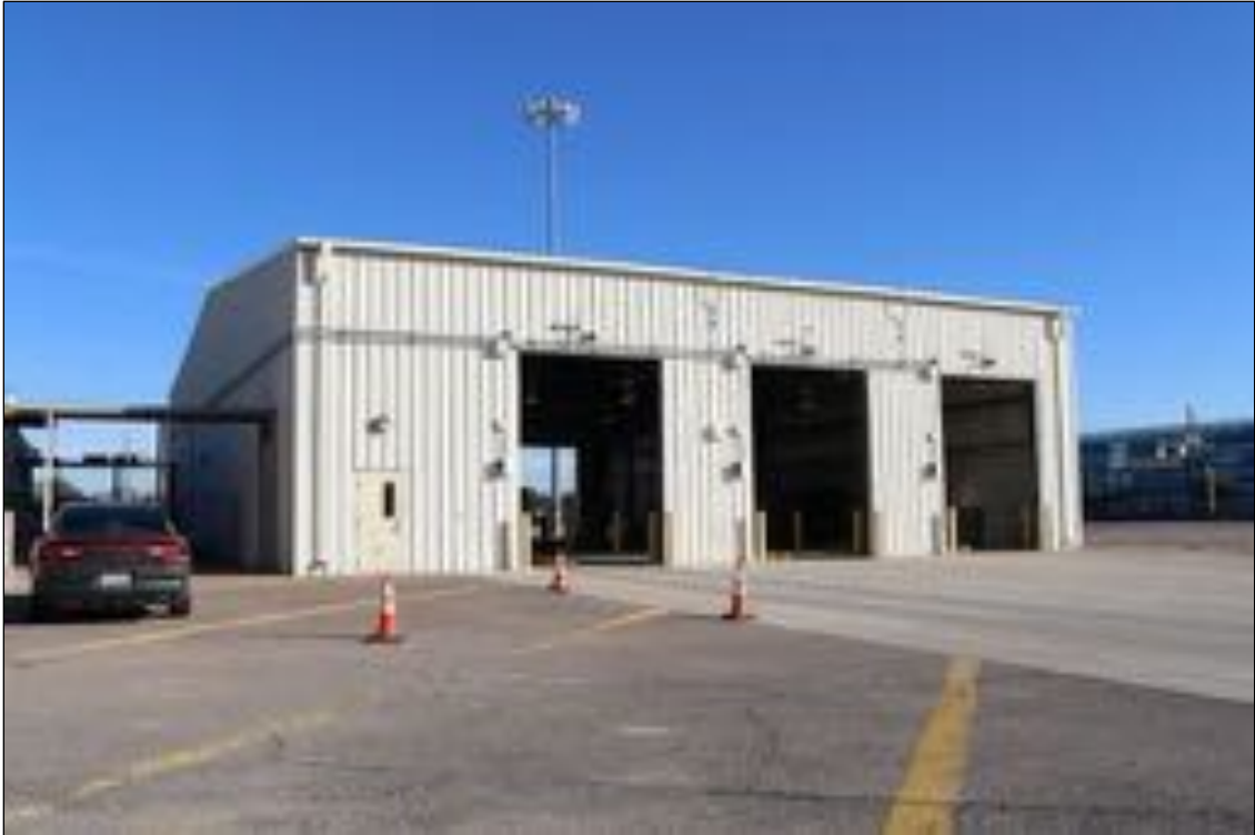
Figure 207. 4000 E Paisano Drive (Inspection Shed), looking northeast.
