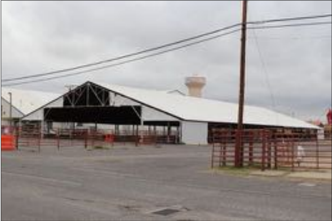
Figure 230. Event Center Shed Structure, looking southeast.
