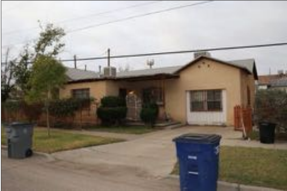
Figure 45. 4030 Laredo Avenue (Residence), looking west.
