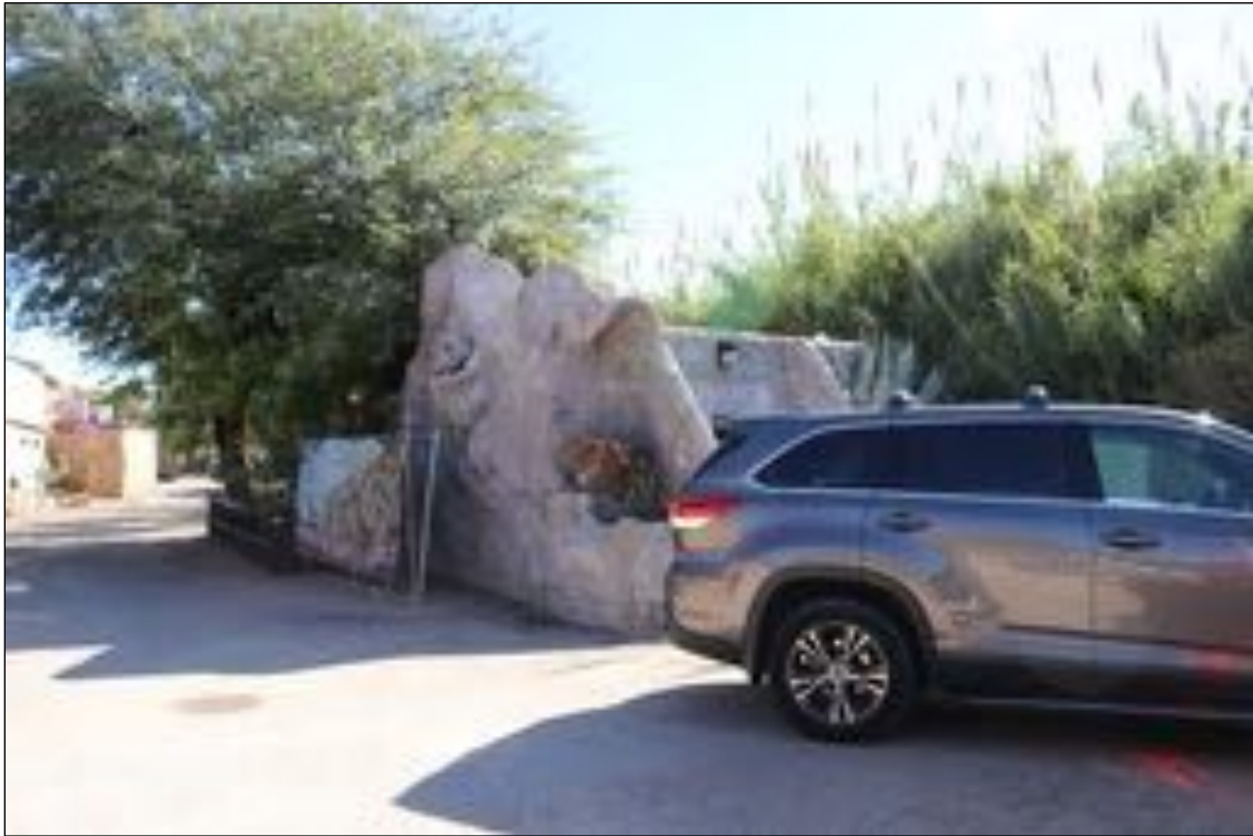
Figure 241. Holding, under construction, looking southeast.
