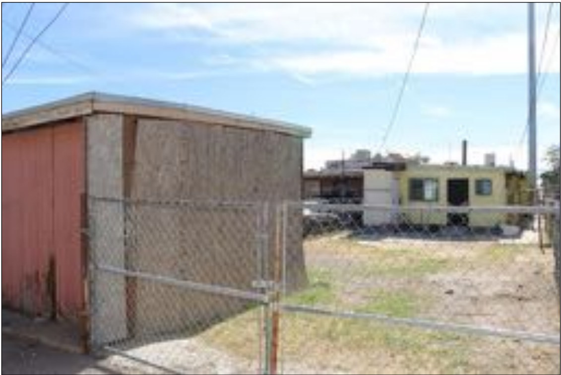
Figure 165. 3819 Findley Avenue (Residence) rear, looking southeast.
