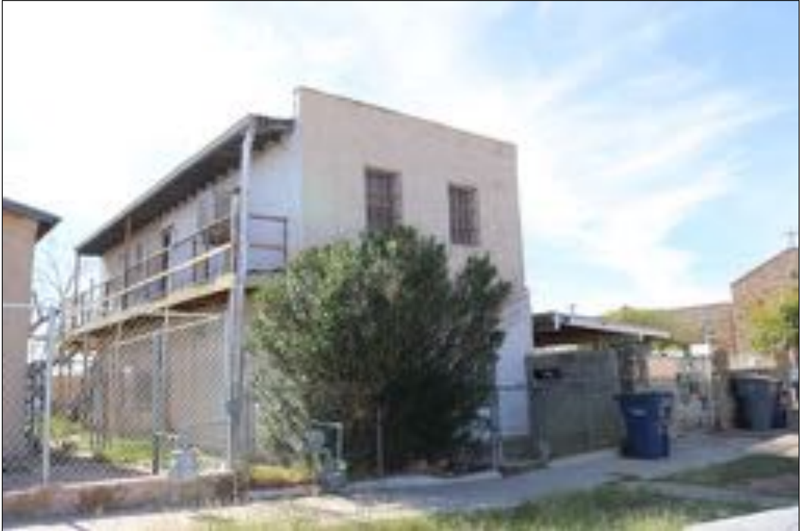
Figure 155. 3810 Findley Avenue (Residence), looking southwest.
