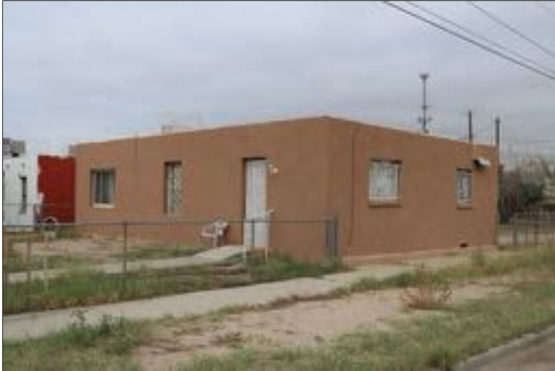
Figure 58. 4019 Oak Court (Residence), looking northwest.
