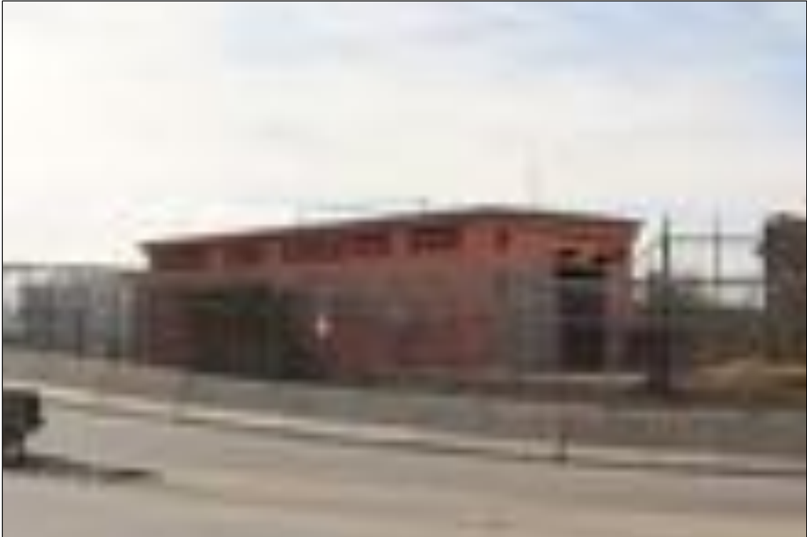
Figure 24. El Paso Water Support Building, looking southwest.
