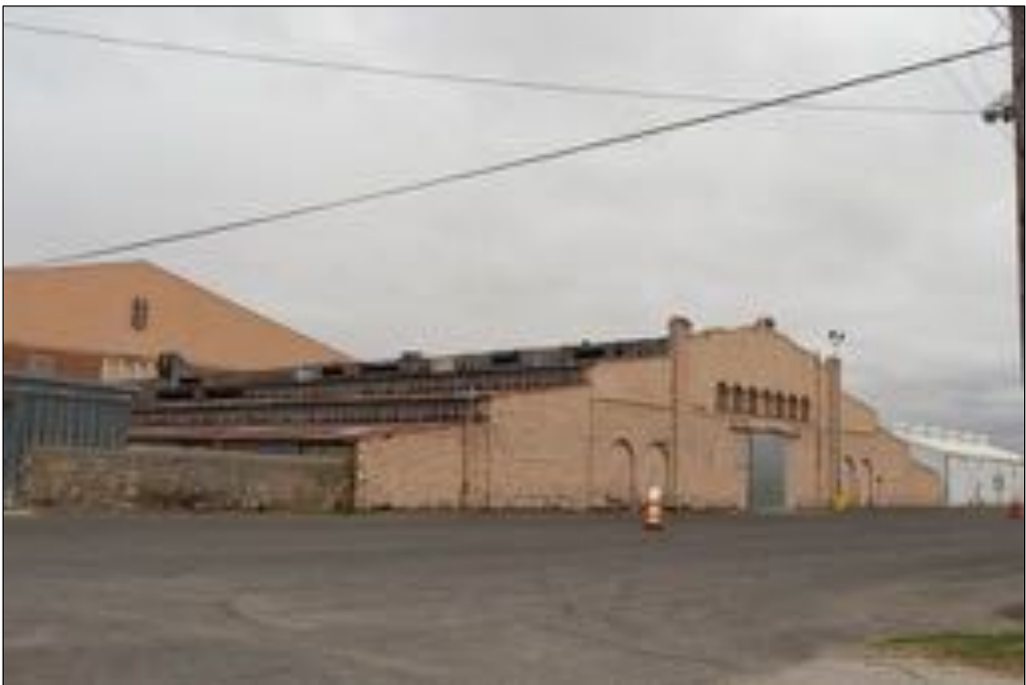
Figure 219. Coliseum Livestock barns, looking northeast.
