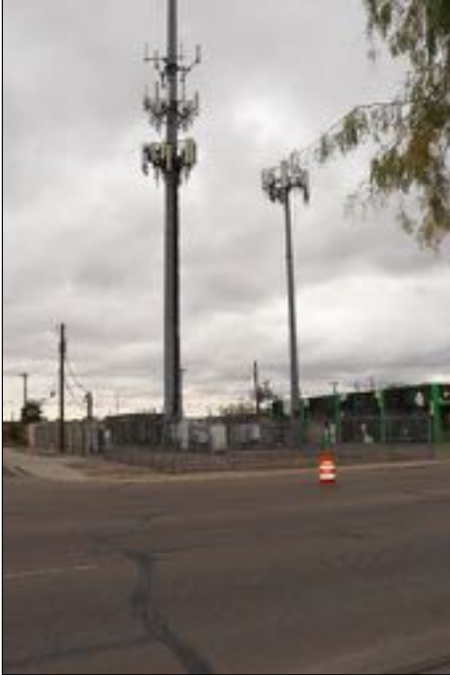
Figure 28. 3930 Delta Drive (Substation), looking southwest.
