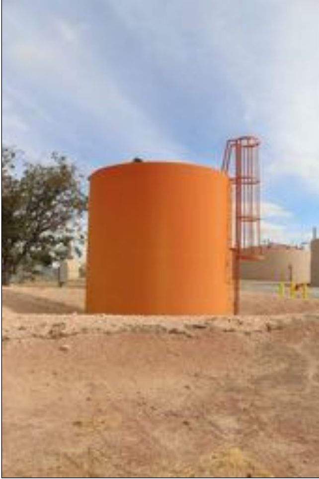
Figure 249. Diesel Tank, 20,000-gallon capacity, looking southeast.
