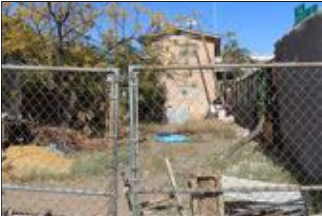
Figure 198. 3826 E San Antonio Avenue (Residence) rear, looking north.
