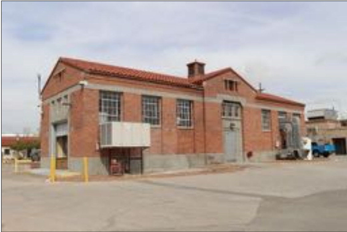
Figure 251. Shop, former Pump House, looking northeast.
