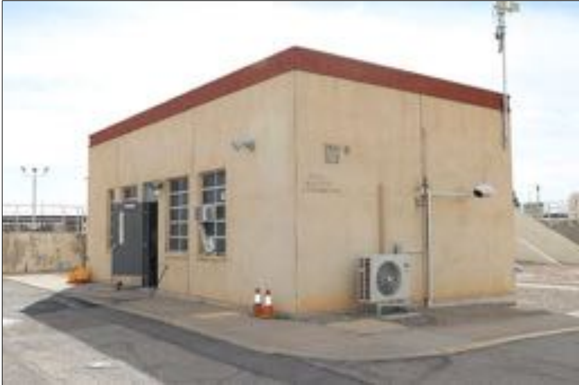
Figure 262. Oxygen Generation Control Building, looking southwest.
