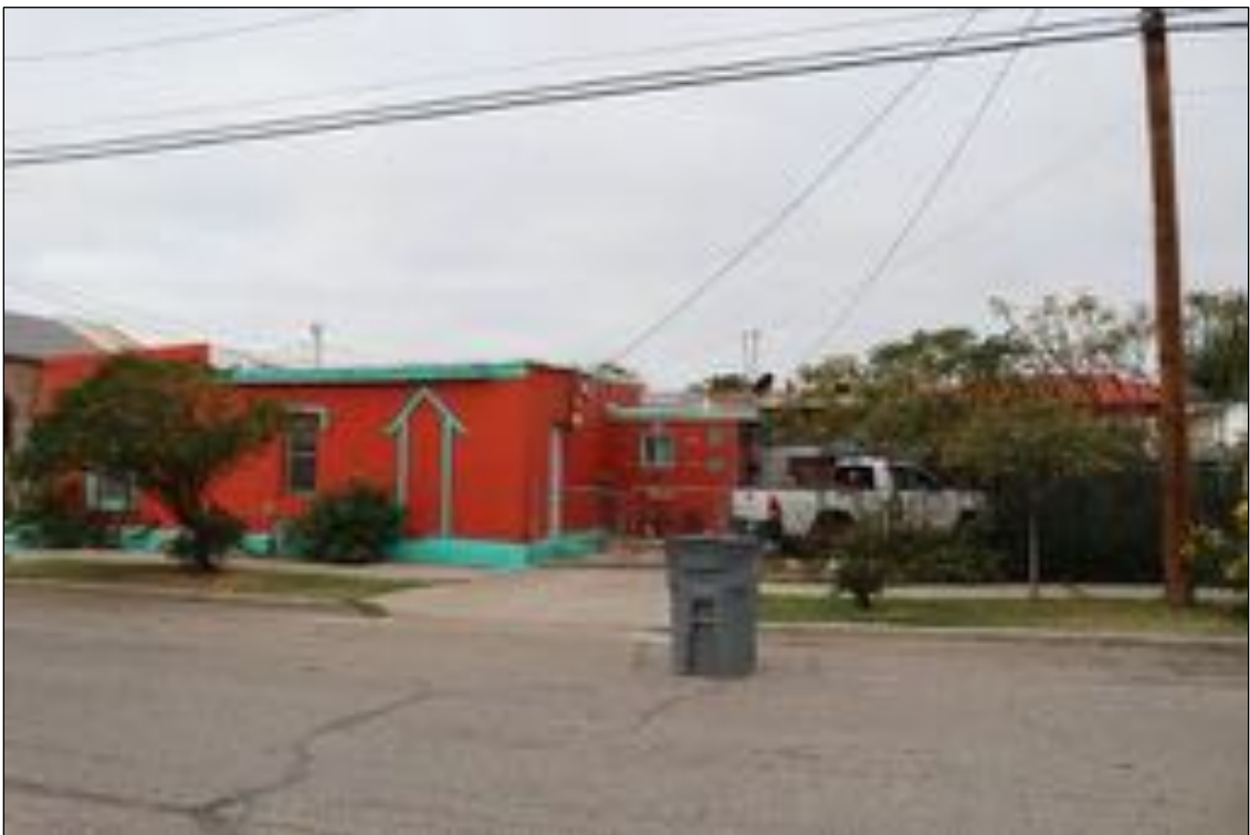
Figure 150. 3737 Findley Avenue (Residence) rear, looking west.
