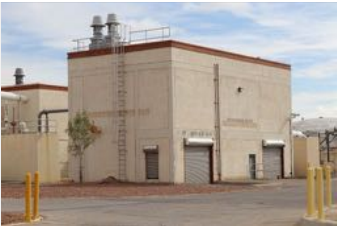
Figure 257. Grit Dewatering Building, looking southeast.
