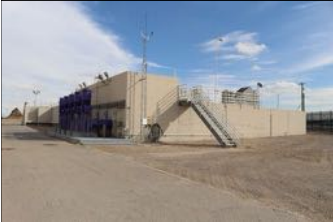
Figure 266. Effluent Pump Station and Filters, looking southeast.
