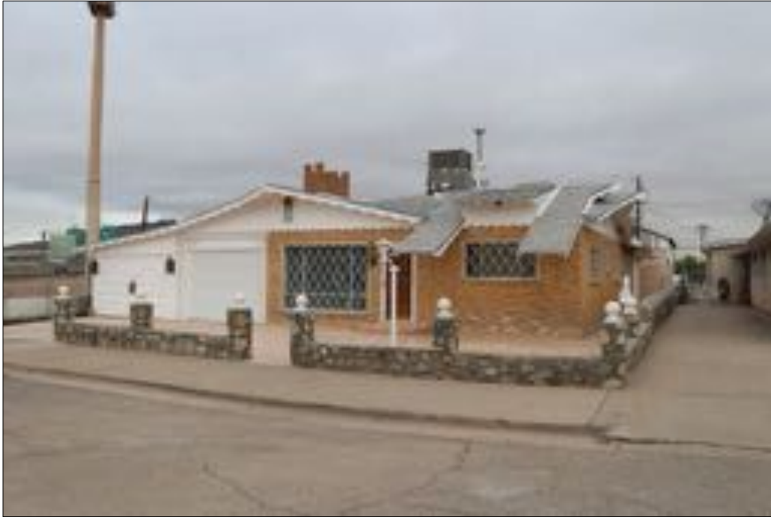
Figure 51. 4003 Oak Court (Residence), looking northwest.
