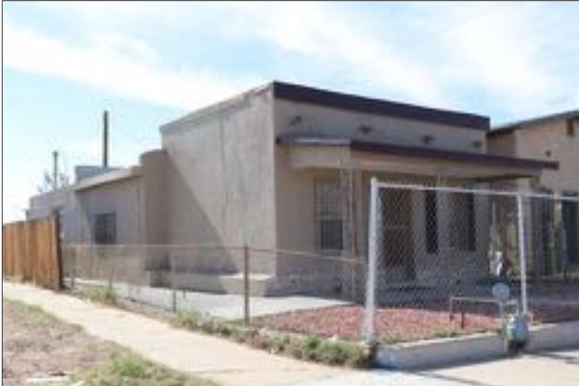
Figure 160. 3816 Findley Avenue (Residence), looking southwest.
