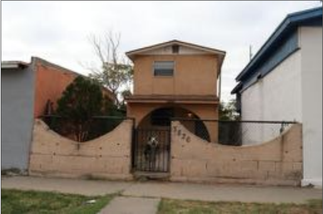
Figure 197. 3826 E San Antonio Avenue (Residence), looking south.
