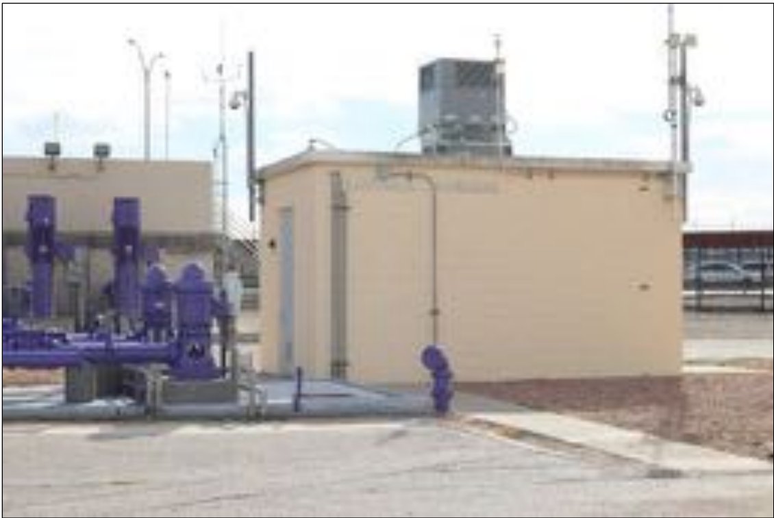
Figure 265. Electrical Building, looking south.
