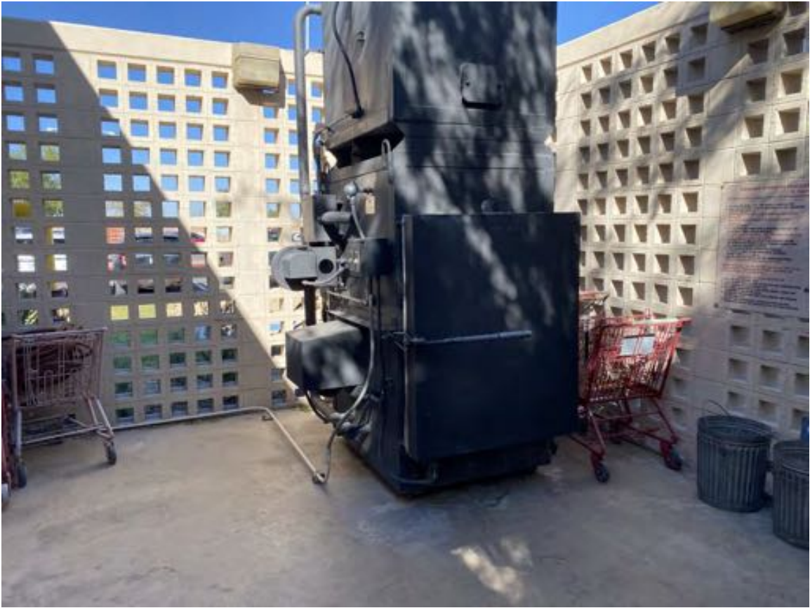
Photograph 31: View looking north of the incinerator.
