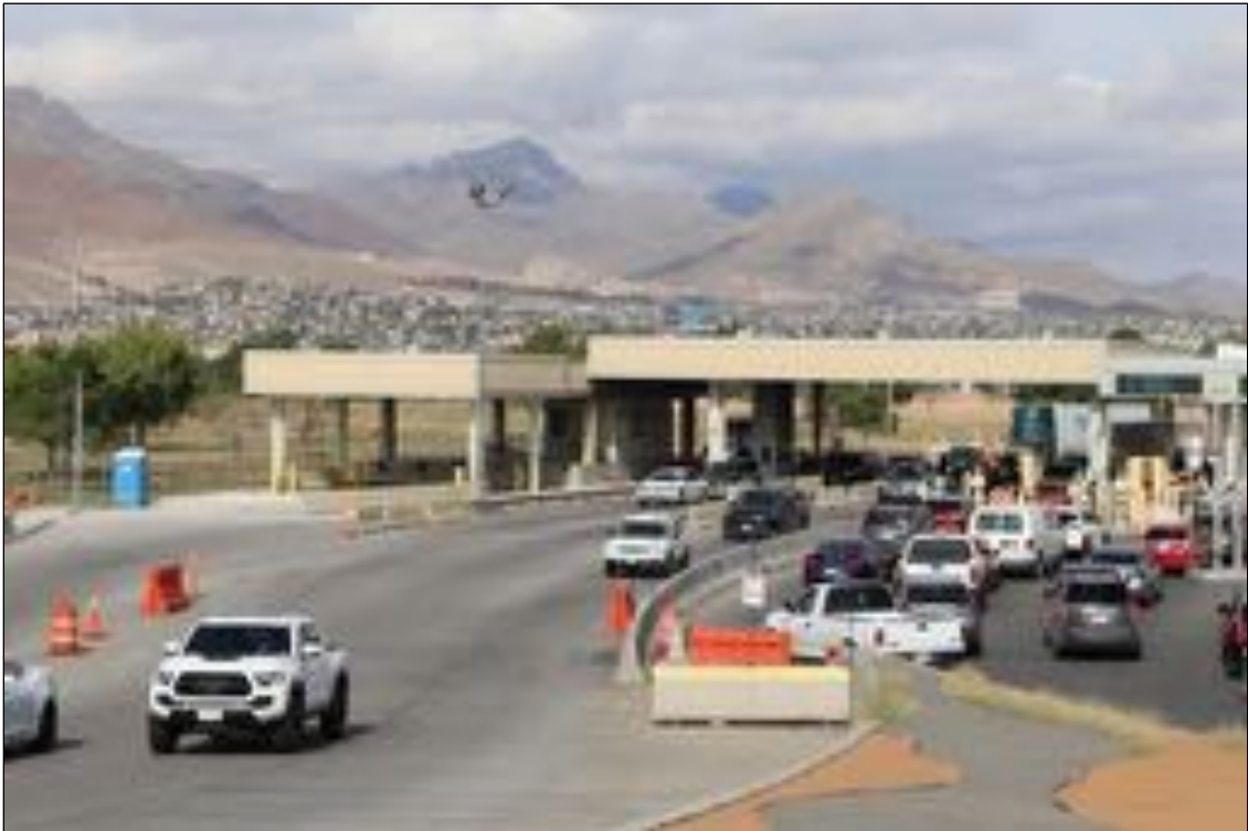
Figure 73. 3600 E Paisano Drive (Southbound Inspection Canopy), looking northwest.
