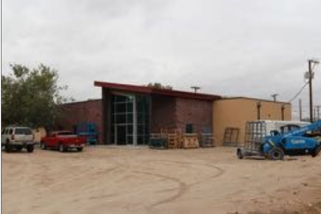
Figure 23. Unnamed El Paso Water Building, looking southeast.
