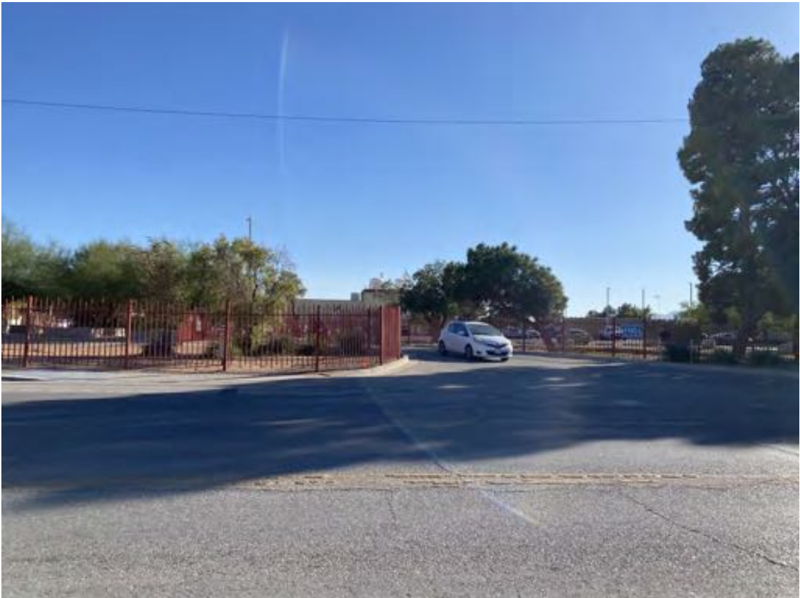
Photograph 20: View looking south across Delta Drive of the Water Treatment Plant south of the County property.
