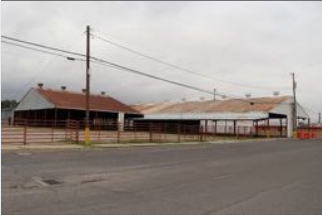
Figure 224. Holding Area Shelter (right) with addition (left), looking southeast.
