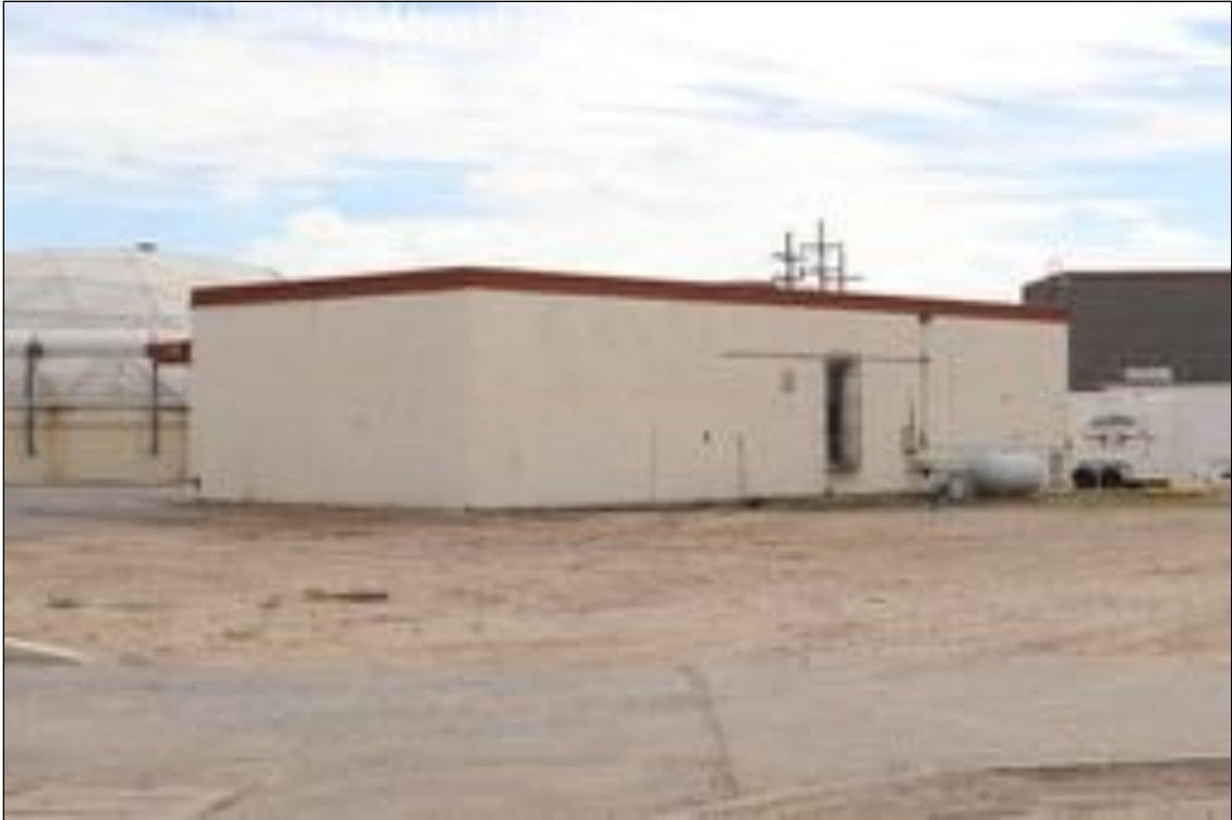
Figure 256. Building, looking southwest.
