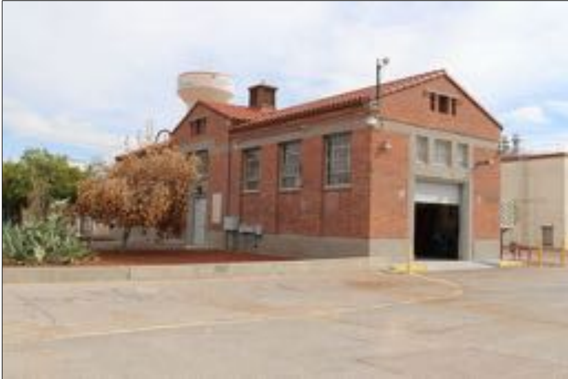
Figure 250. Shop, former Pump House, looking southeast.
