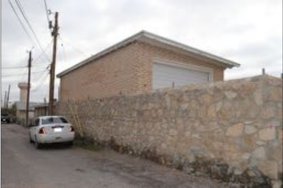
Figure 52. 4001 Oak Court (Garage) associated with 4003 Oak Court, looking southeast.
