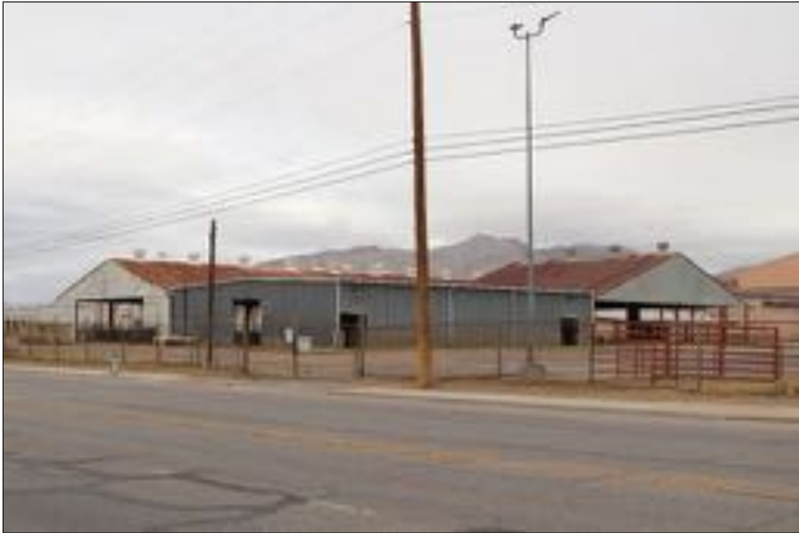
Figure 229. Holding Area Storage Building (right) and Holding Area Shelter (left and background), looking northwest.
