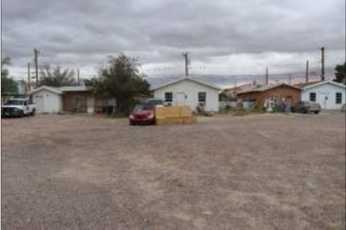
Figure 44. 4019 Laredo Avenue (Residence), looking north. Note from left to right units A, B, C, and D.
