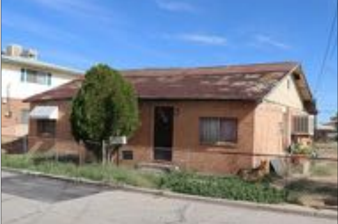
Figure 109. 226 Hardesty Place (Residence), looking northeast.
