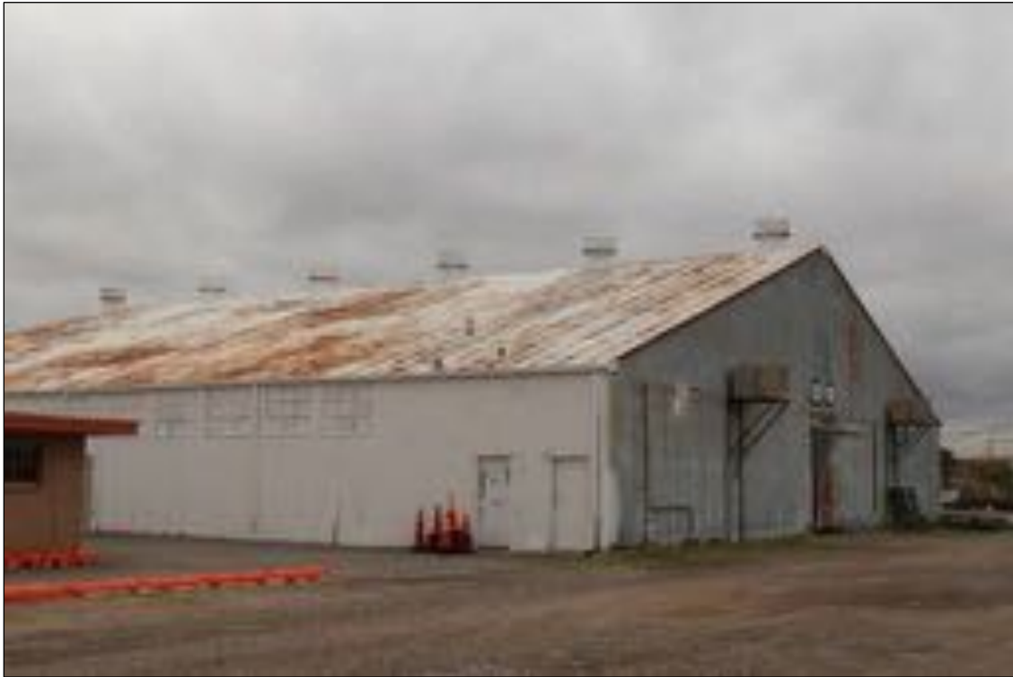
Figure 226. Holding Area Shelter, western wing, looking southeast.
