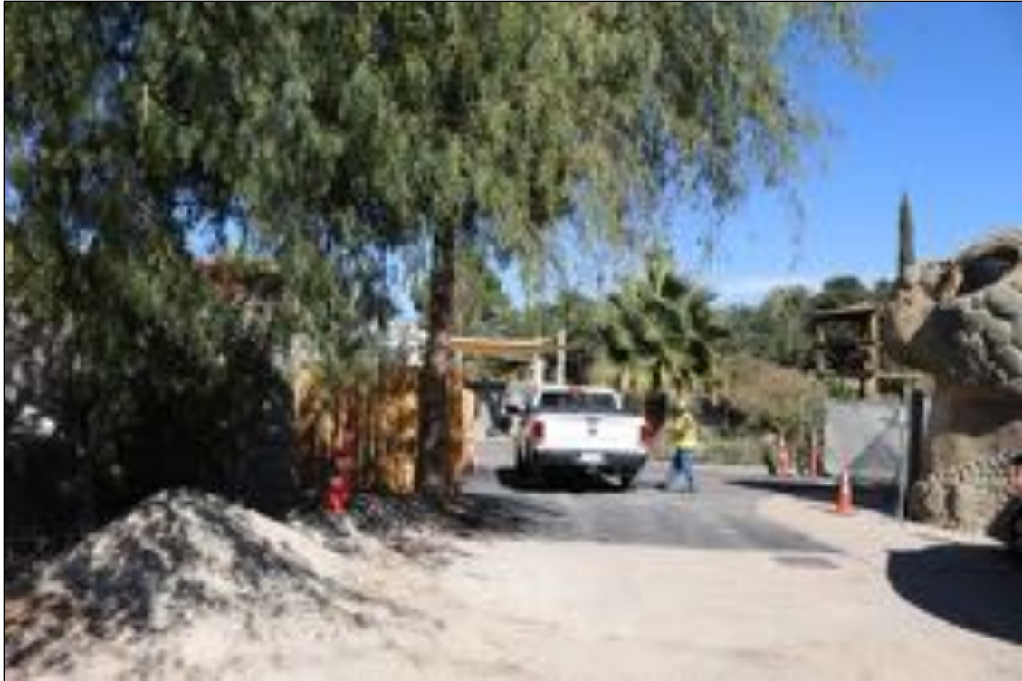
Figure 240. Holding, under construction, looking southwest.
