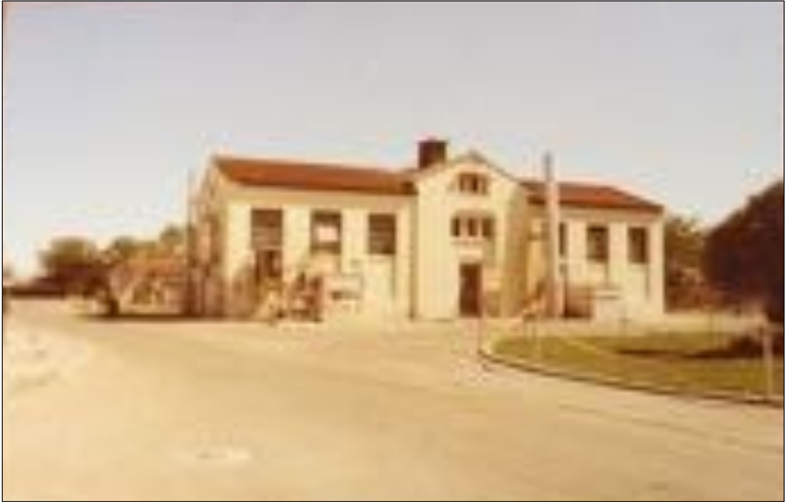
Figure 252. Shop, former Pump House, historic photograph ca. 1943, looking southwest.
