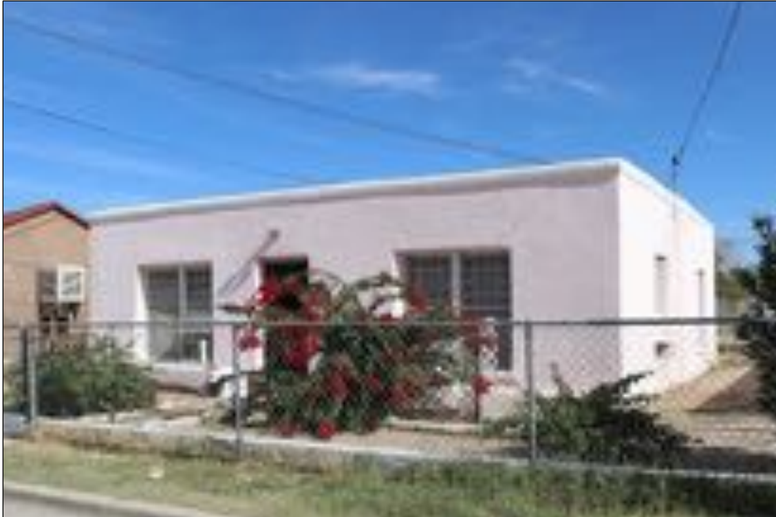
Figure 92. 210 Hardesty Place (Residence), looking northeast.
