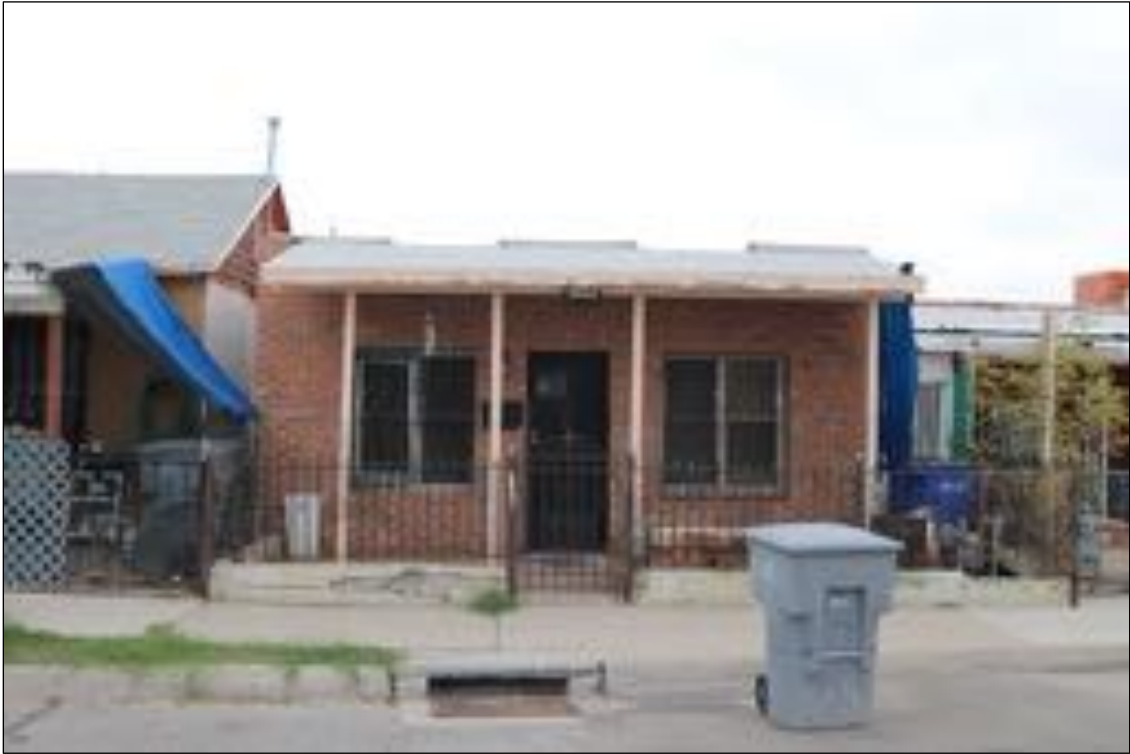
Figure 178. 3722 E San Antonio Avenue (Residence), looking south.
