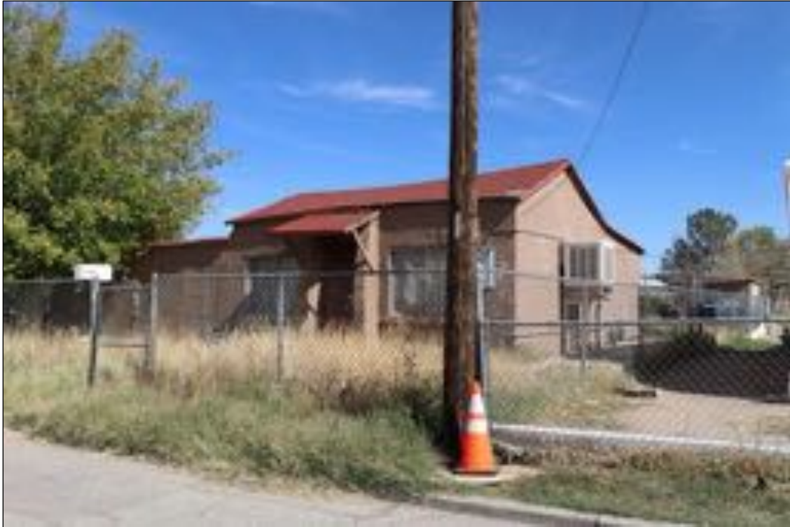
Figure 89. 208 Hardesty Place (Residence), looking northeast.
