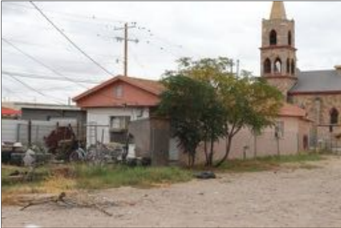
Figure 146. 3733 Findley Avenue (Residence) rear, looking southeast.
