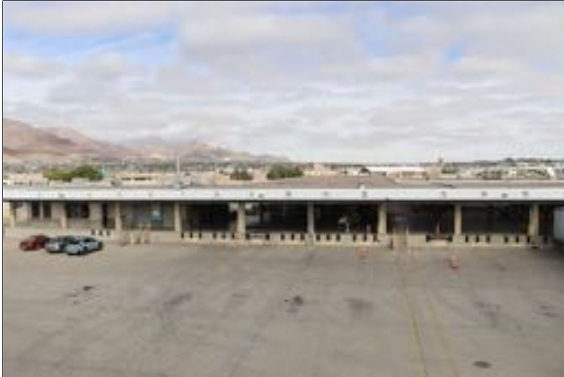
Figure 106. 3600 E Paisano Drive (Building D Cargo Building Dock), looking northwest.
