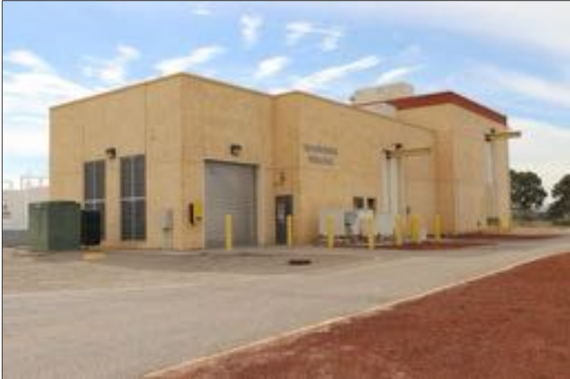
Figure 254. Headworks Building, looking southwest.
