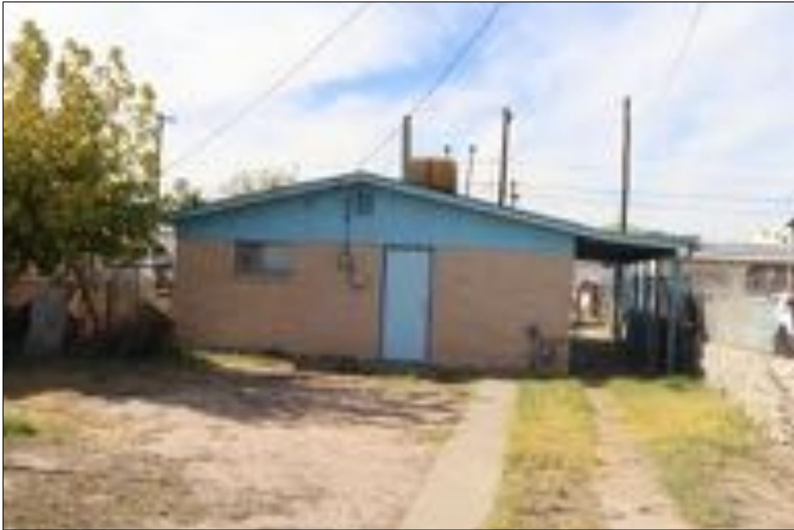
Figure 98. 214 Hardesty Place (Residence) rear, looking west.
