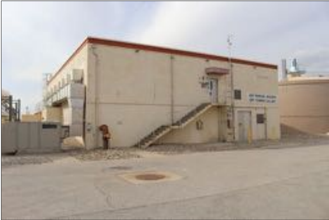
Figure 267. Grit Building, looking northwest.
