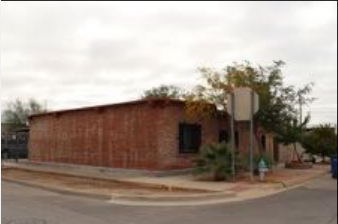
Figure 186. 3800 E San Antonio Avenue (Residence), looking southeast.
