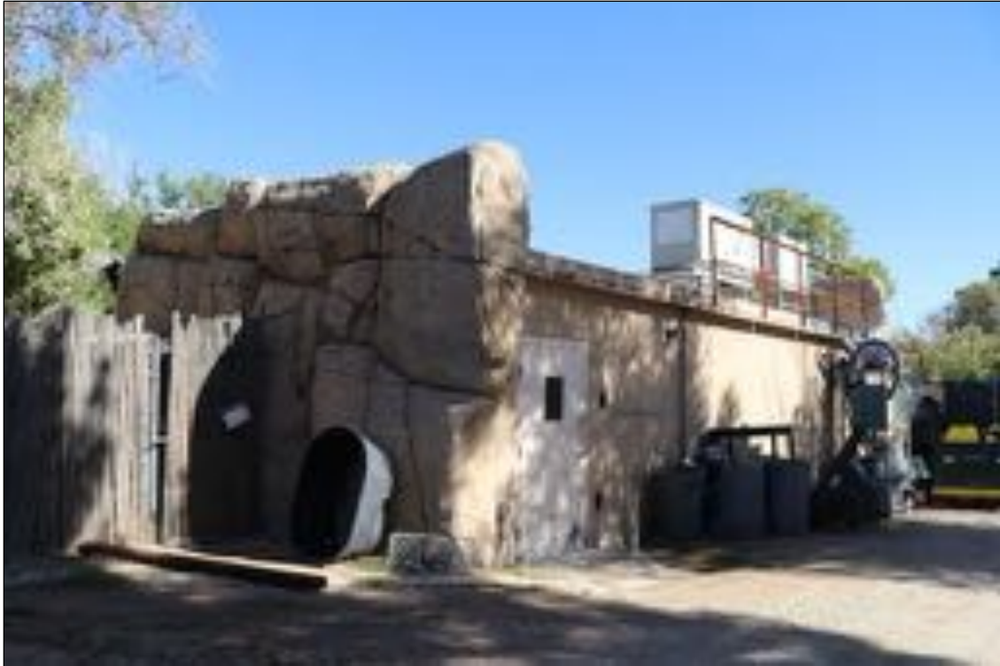
Figure 245. Malayan Tapir Housing, looking northeast.
