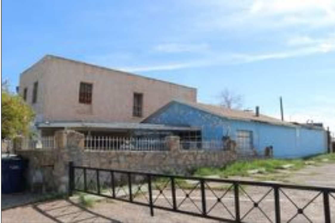
Figure 151. 3808 Findley Avenue (Residence), looking southeast.
