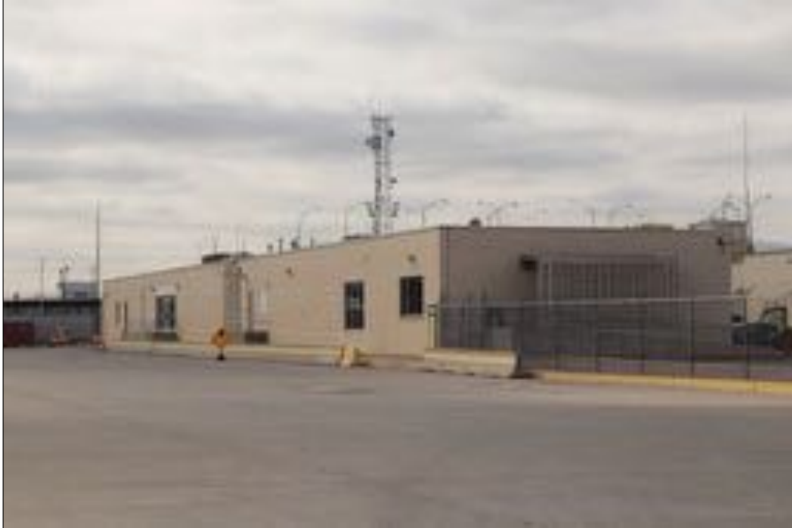
Figure 51. 3600 E Paisano Drive (Building B Administration Building), looking southwest.
