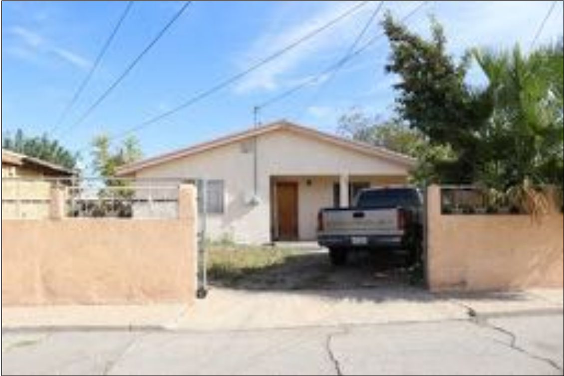
Figure 85. 202 Hardesty Place (Residence), looking east.
