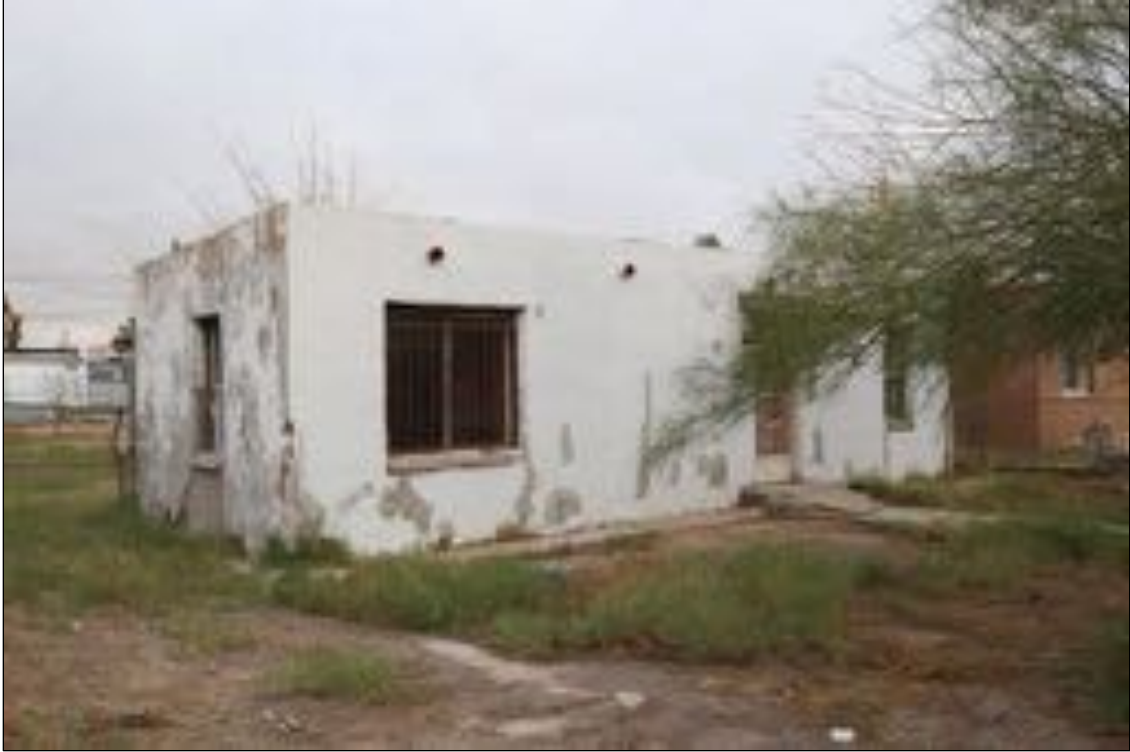
Figure 57. 4007 Oak Court (Residence), looking northeast.
