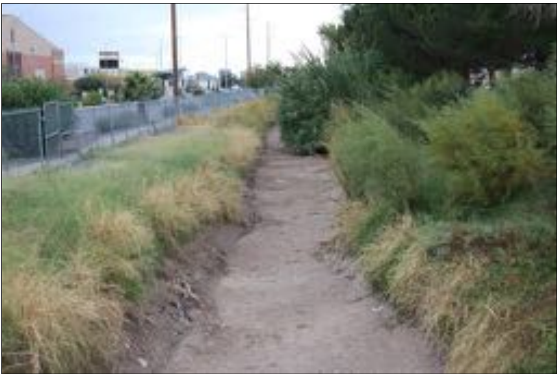
Figure 8. Franklin Canal, along Paisano Drive, looking west.
