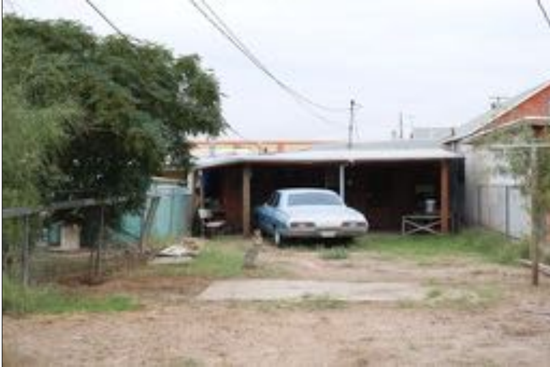
Figure 179. 3722 E San Antonio Avenue (Residence) rear, looking north.
