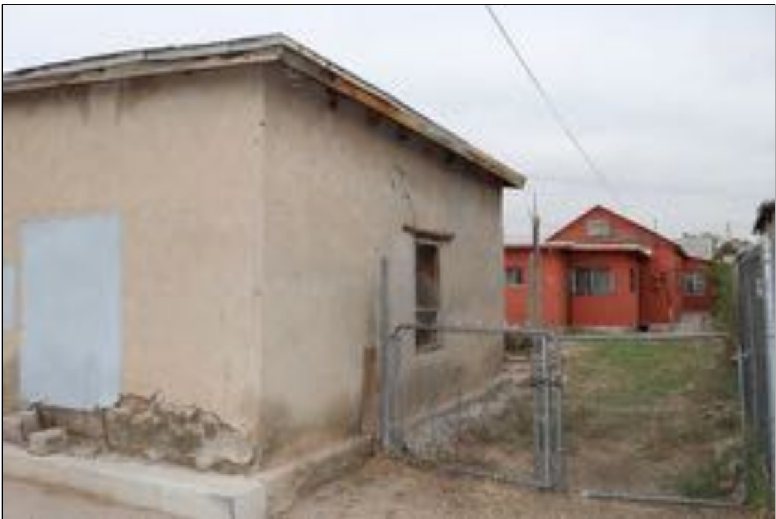
Figure 181. 3724 E San Antonio Avenue (Residence) rear, looking north.
