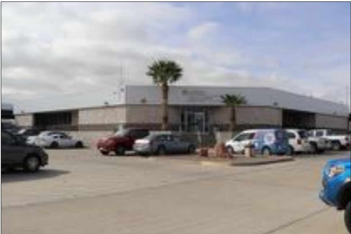
Figure 95. 3600 E Paisano Drive (Building D Cargo Building), looking southwest.
