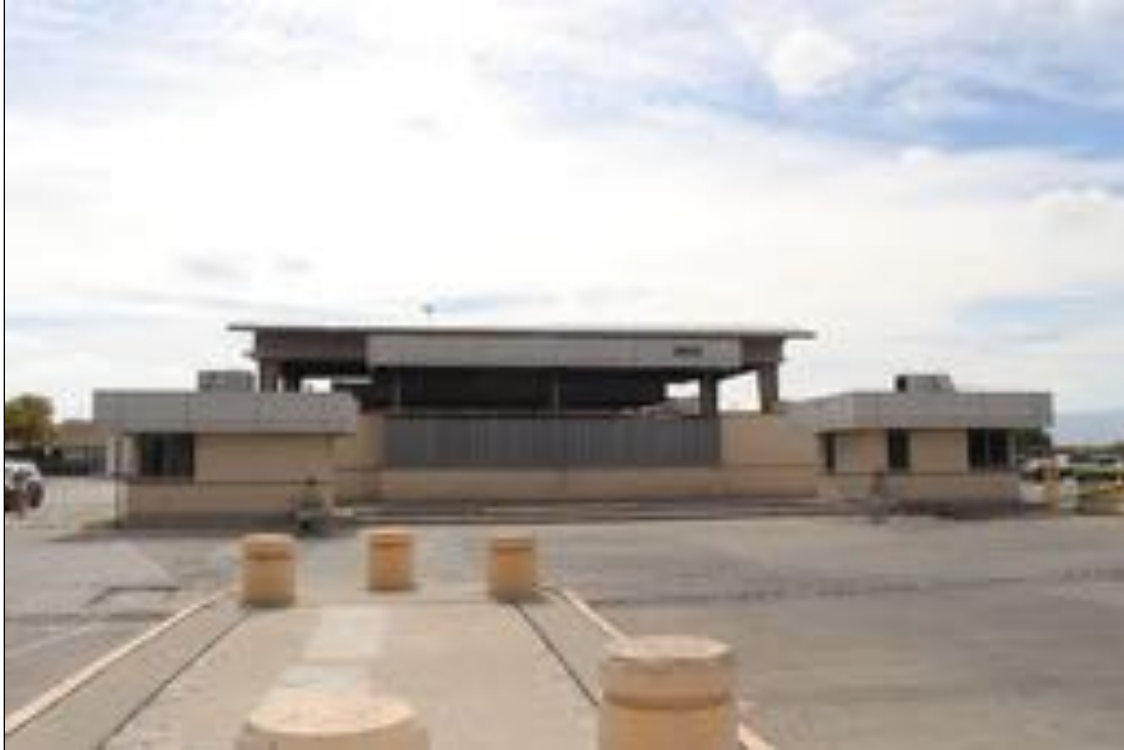
Figure 62. 3600 E Paisano Drive (Building C Head House and TAC Booths), looking southwest.
