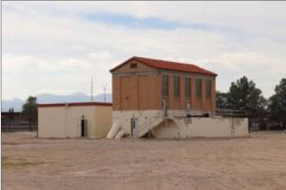
Figure 258. Building, looking southwest.
