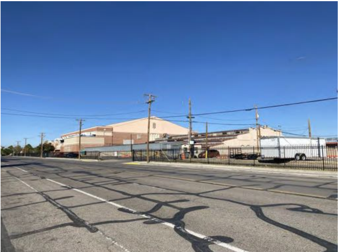
Photograph 12: View looking northeast of the El Paso County Coliseum on the County property east of the TxDot property.
