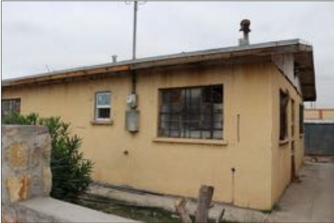
Figure 172. 3706 E San Antonio Avenue (Residence) rear, looking north.
