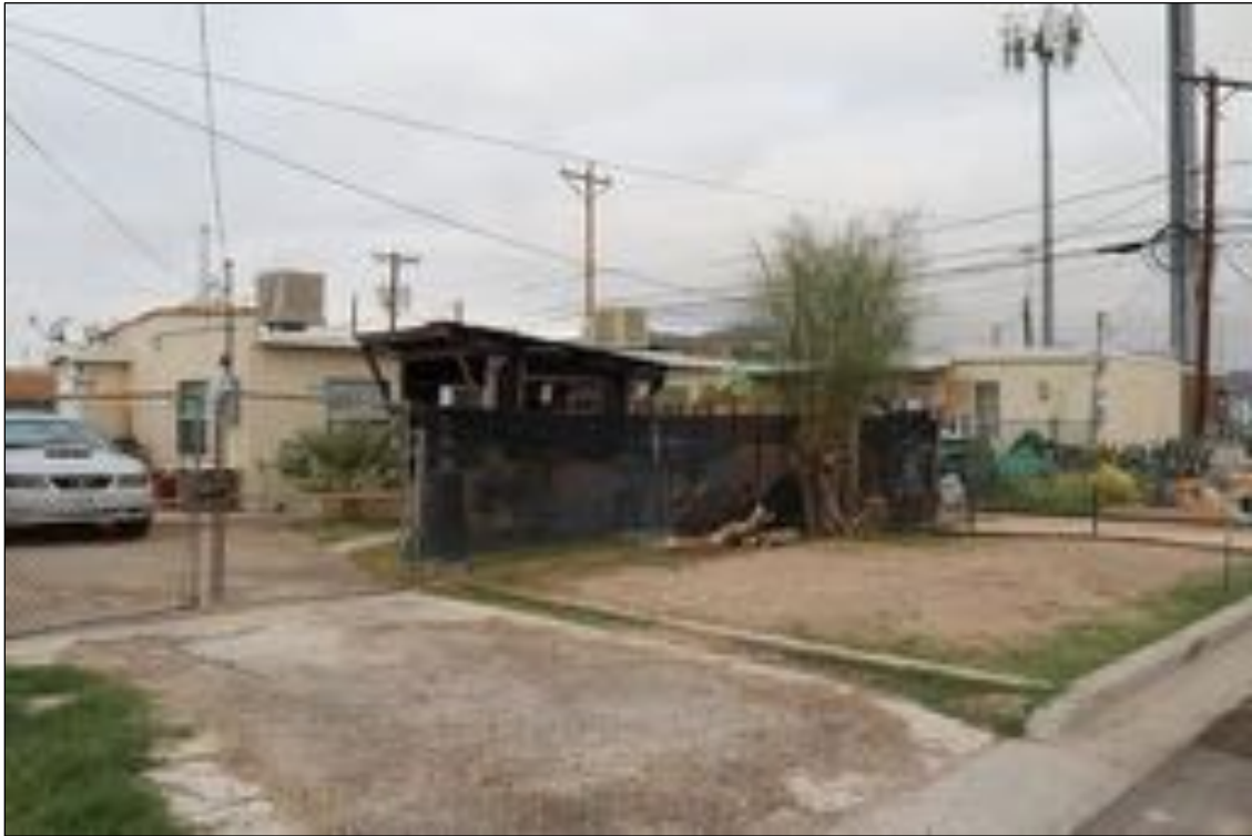
Figure 37. 3923 Laredo Avenue (Residence) rear, looking northwest.
