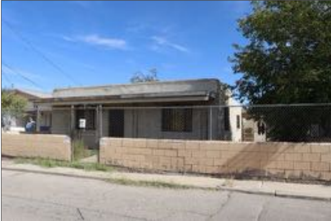
Figure 86. 204 Hardesty Place (Residence), looking northeast.
