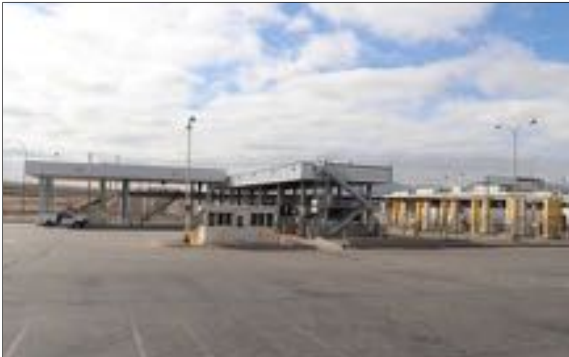
Figure 714. 3600 E Paisano Drive (Inbound Commercial Primary Inspection Canopy with Booth and Empty Truck Canopy), Empty Truck Canopy (left), Inbound Commercial Primary Inspection Canopy (right) and Booth (foreground), looking south.
