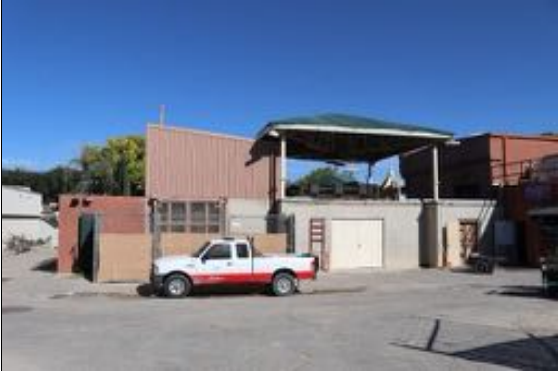
Figure 244. Elephant Barn Complex, looking north.
