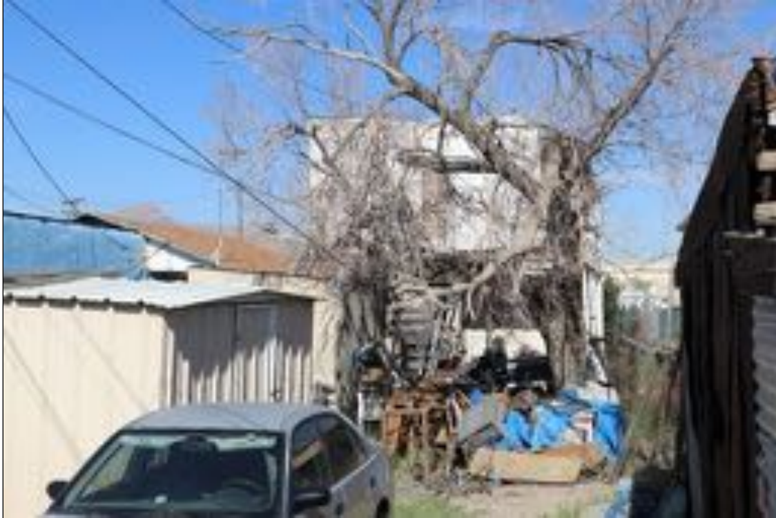
Figure 156. 3810 Findley Avenue (Residence) rear, looking north.
