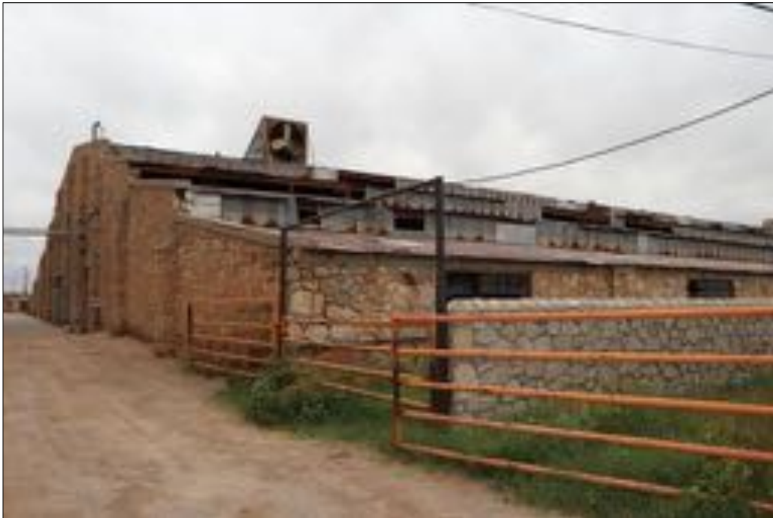
Figure 217. Coliseum Livestock barns, looking east.
