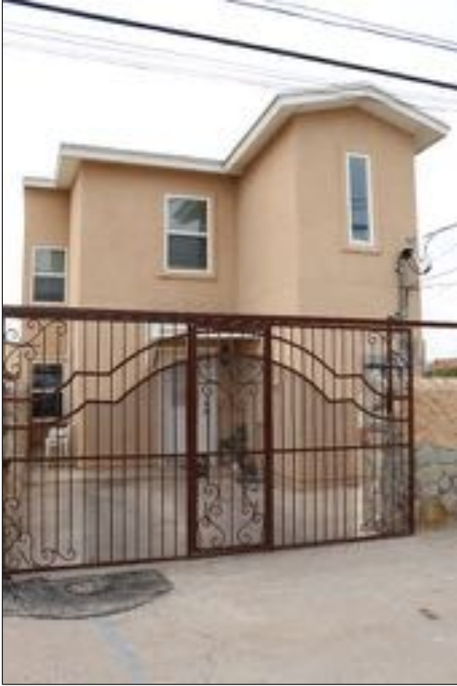
Figure 136. 3711 Findley Avenue (Residence) rear, looking south.
