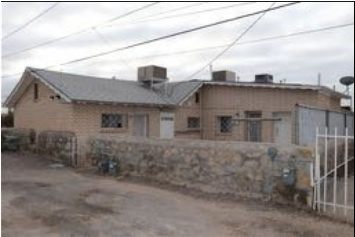
Figure 55. 4005 Oak Court (Residence) rear, looking southeast.
