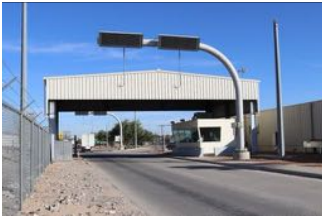
Figure 209. 4000 E Paisano Drive (Exit Booth), looking north.
