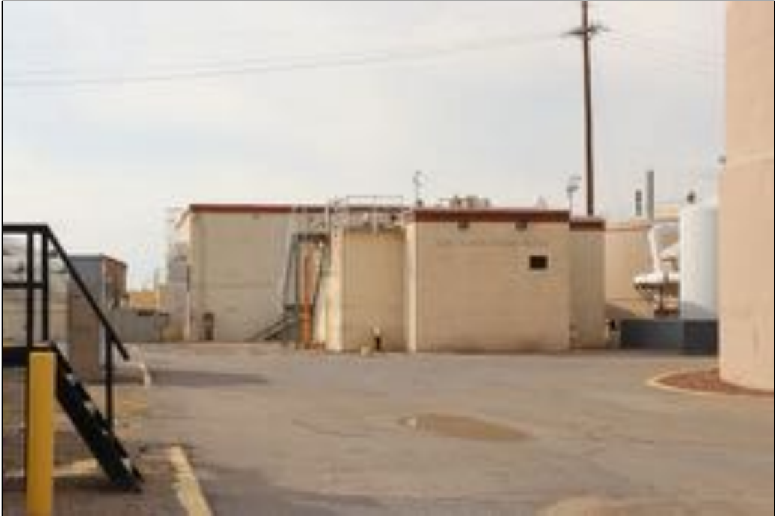
Figure 268. Mixed Sludge Pumping Station, looking west.
