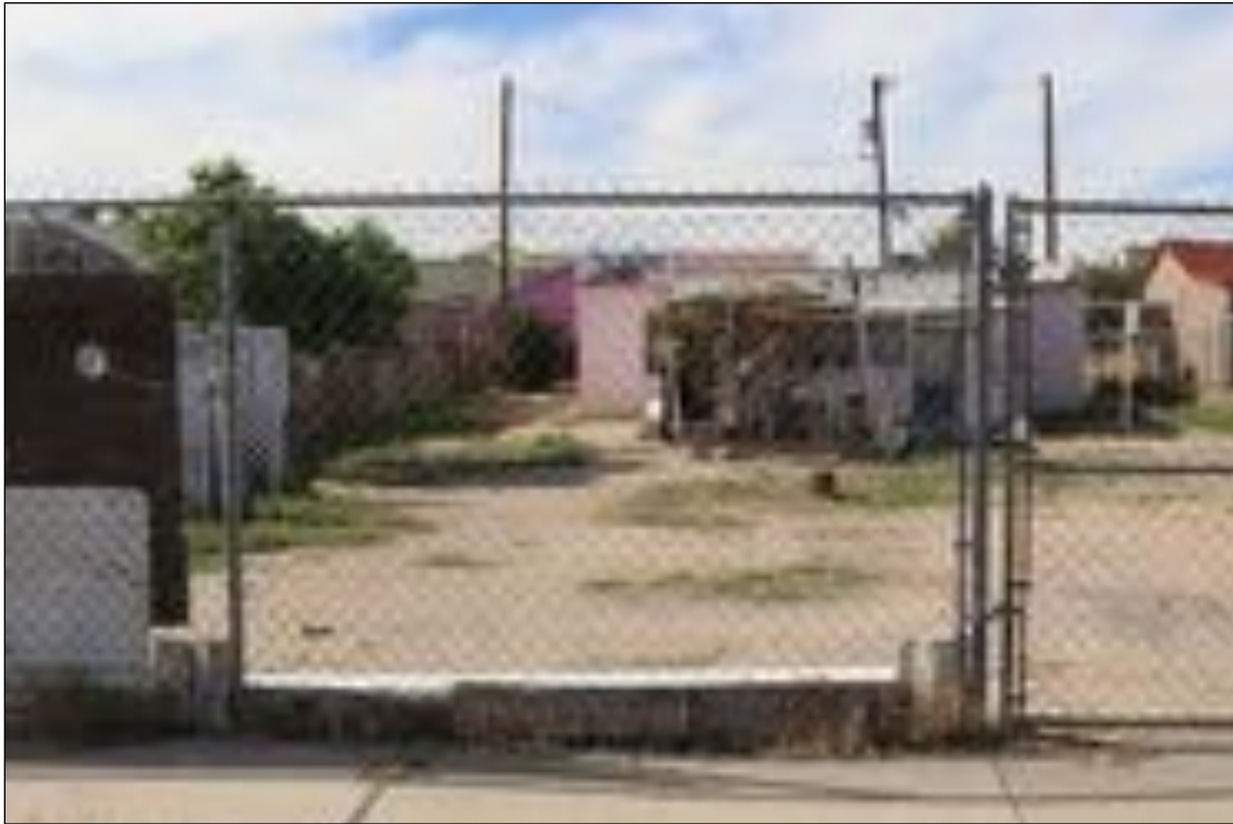
Figure 93. 210 Hardesty Place (Residence) rear, looking west.
