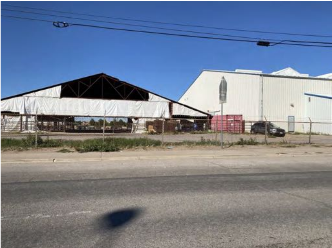
Photograph 14: View looking north of a livestock building and the events center/hockey rink on the County property.
