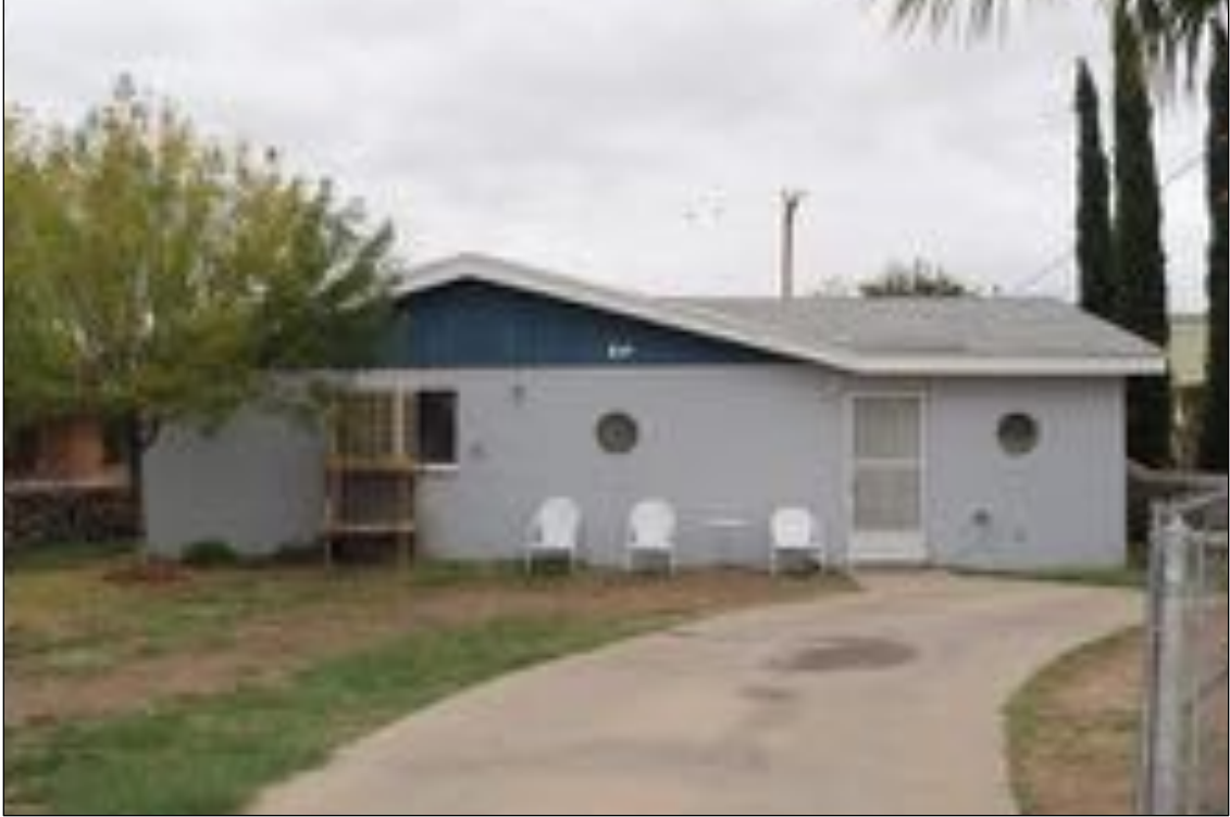
Figure 101. 217 Hardesty Place (Residence), looking west.
