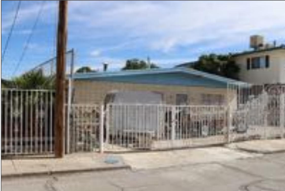
Figure 106. 222 Hardesty Place (Residence), looking east.
