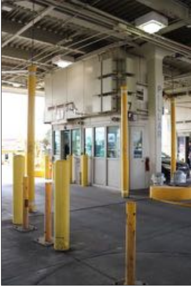
Figure 128. 3600 E Paisano Drive (Building K Primary/Secondary Inspection Canopy), Primary Inspection Canopy booth, looking southwest.
