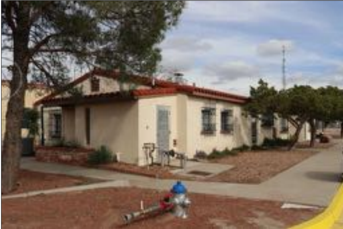
Figure 248. Office, looking northwest.
