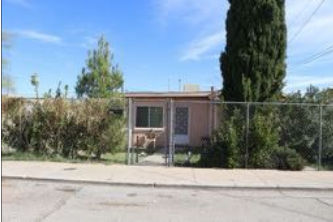
Figure 102. 218 Hardesty Place (Residence), looking east.
