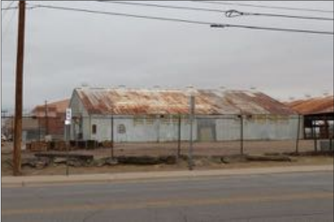
Figure 227. Holding Area Shelter, western wing, looking north.
