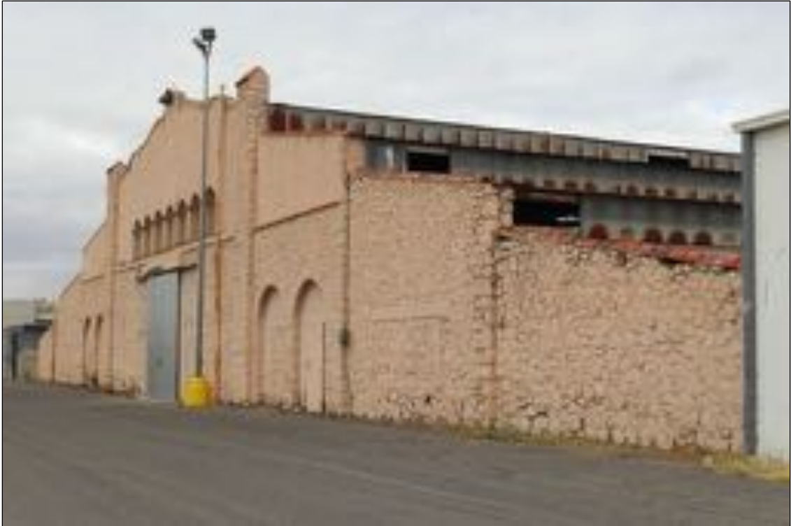
Figure 218. Coliseum Livestock barns, looking northwest.
