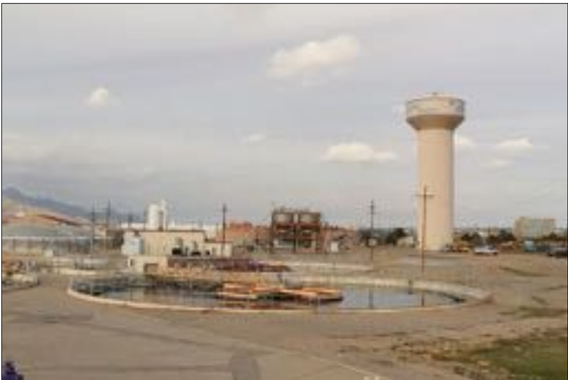
Figure 269. Basins and water tower, looking north.
