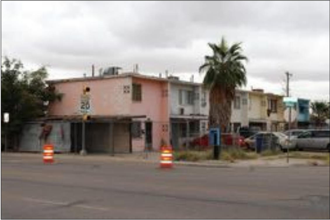
Figure 47. 700–714 S Martinez Street (Apartment Complex), looking southeast.
