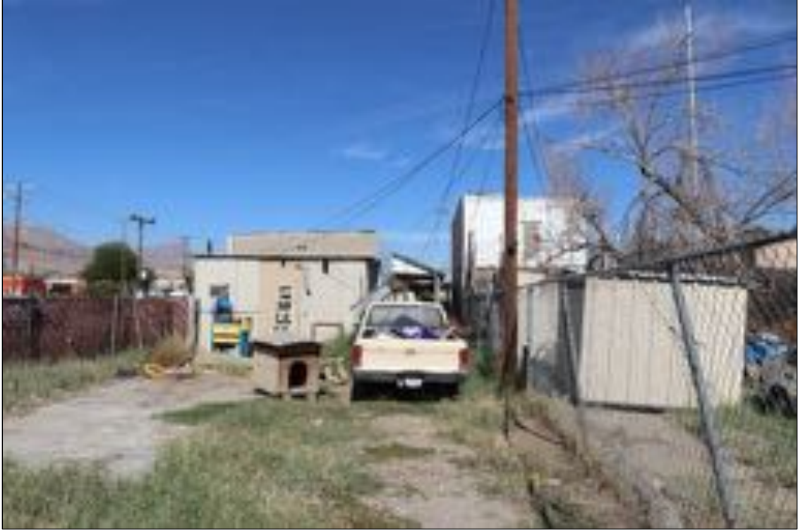
Figure 152. 3808 Findley Avenue (Residence) rear, looking north.
