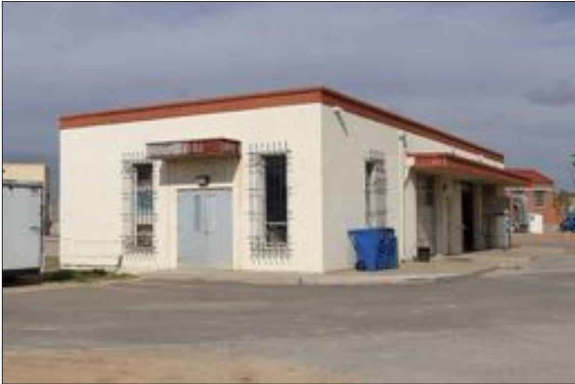
Figure 259. Electrical Shop, looking north.
