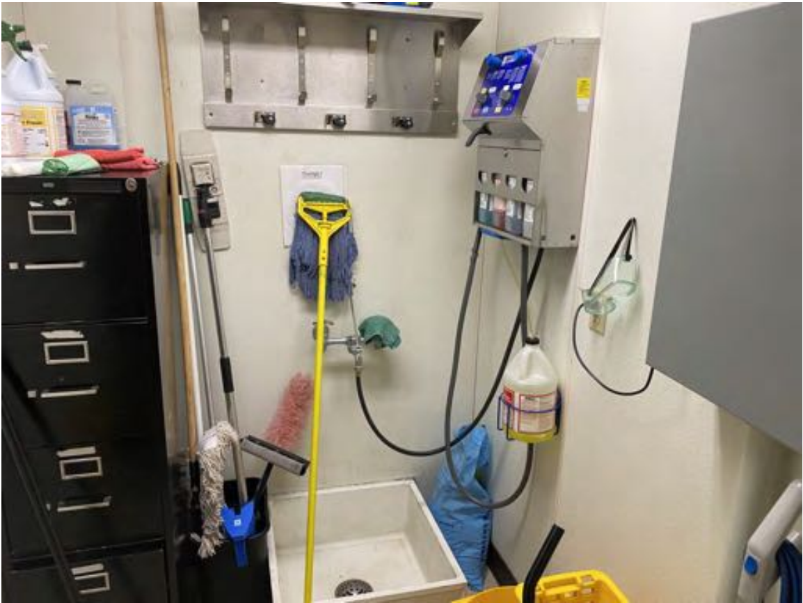
Photograph 23: View of cleaning chemicals in the janitor closet.
