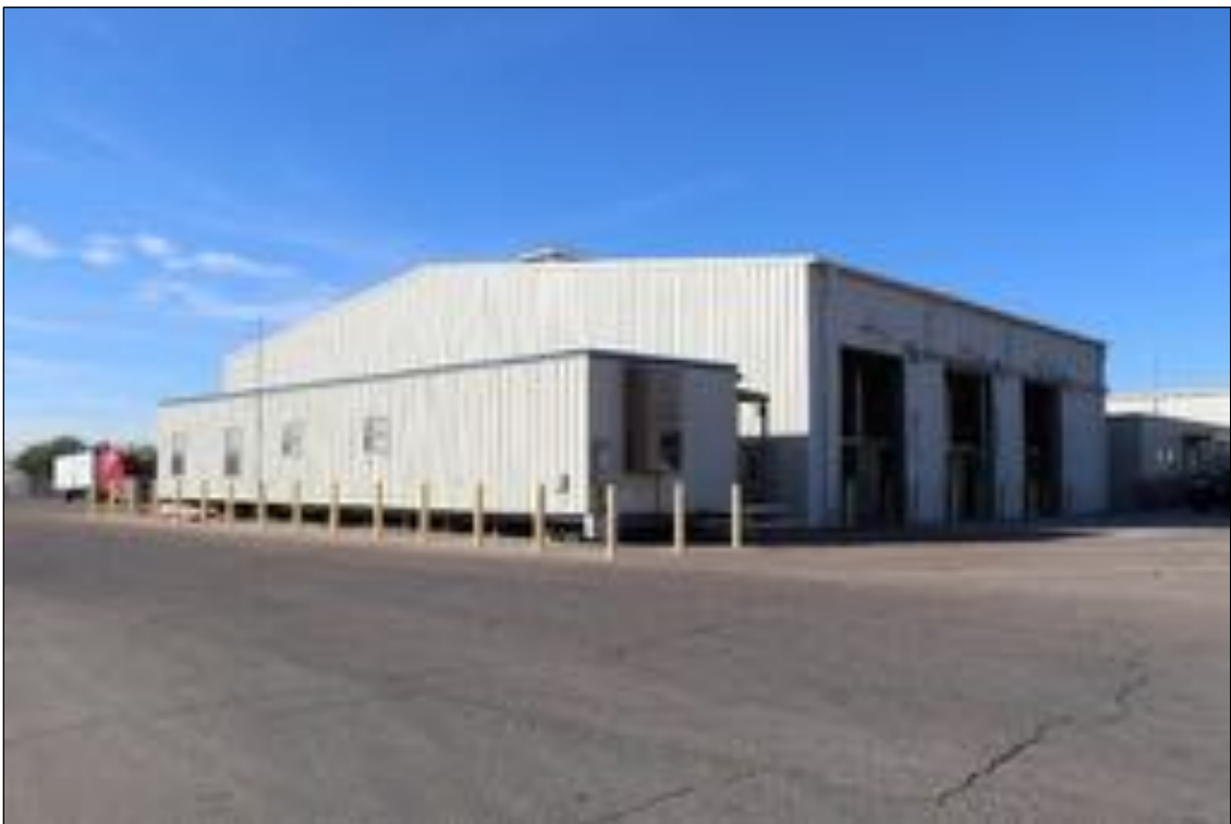
Figure 208. 4000 E Paisano Drive (Inspection Shed), looking southwest.
