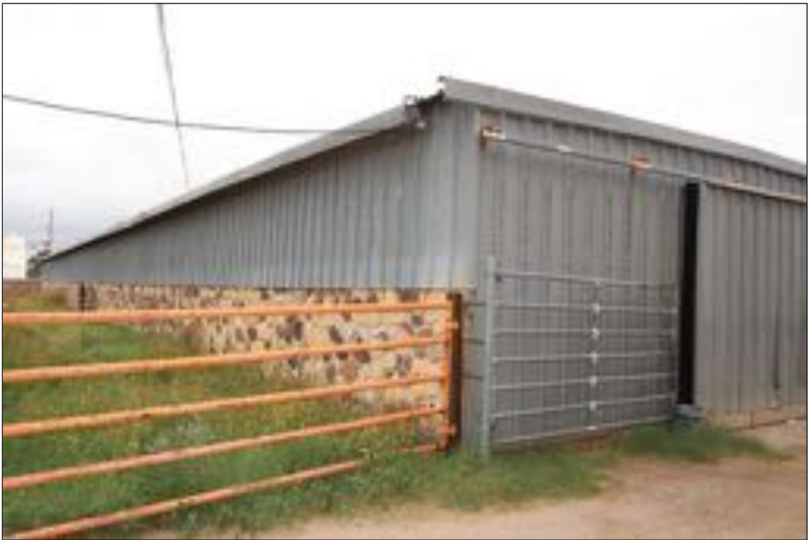
Figure 216. Livestock Barn, looking south.
