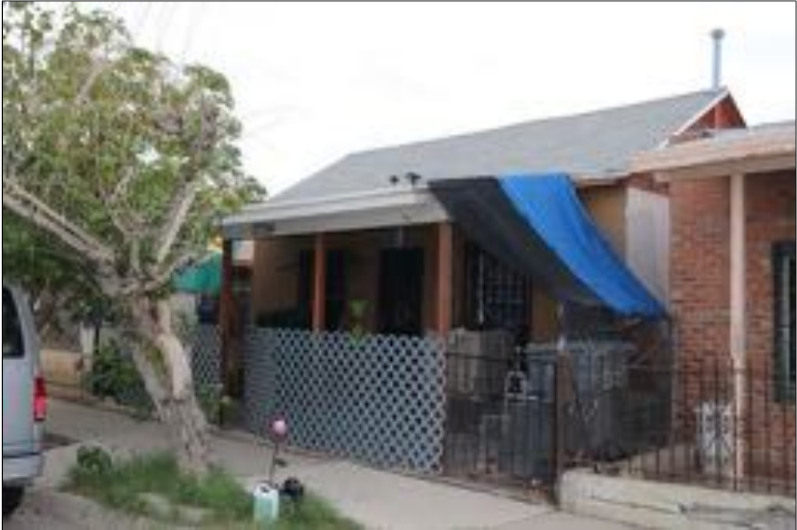
Figure 180. 3724 E San Antonio Avenue (Residence), looking south.
