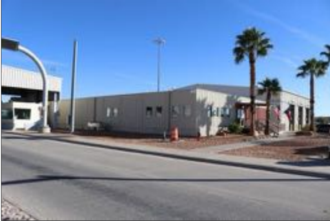
Figure 206. 4000 E Paisano Drive (Office) with inspection shed in the background, looking northeast.
