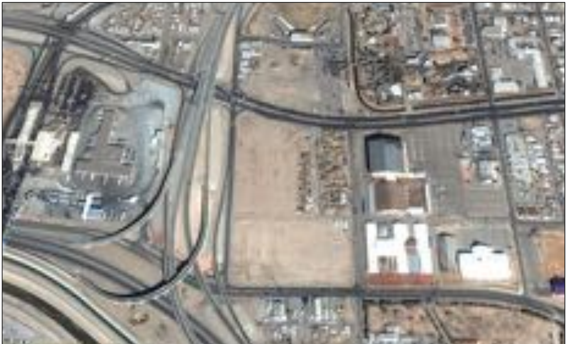
Figure 202. Aerial showing the location of the TxDOT Facility in February 2000 (courtesy of Google Earth).
