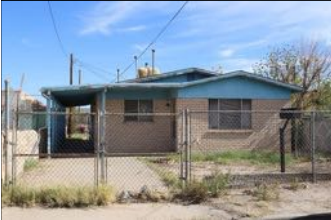
Figure 97. 214 Hardesty Place (Residence), looking east.
