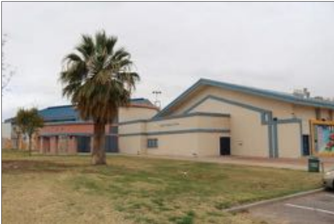
Figure 14. 4321 Delta Drive (Acosta Sports Center), looking northwest.
