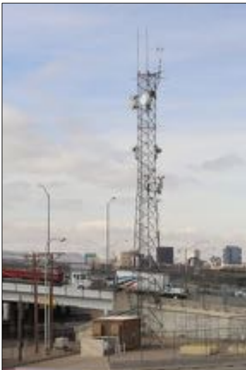
Figure 75. 3600 E Paisano Drive (RVSS Tower), looking west.
