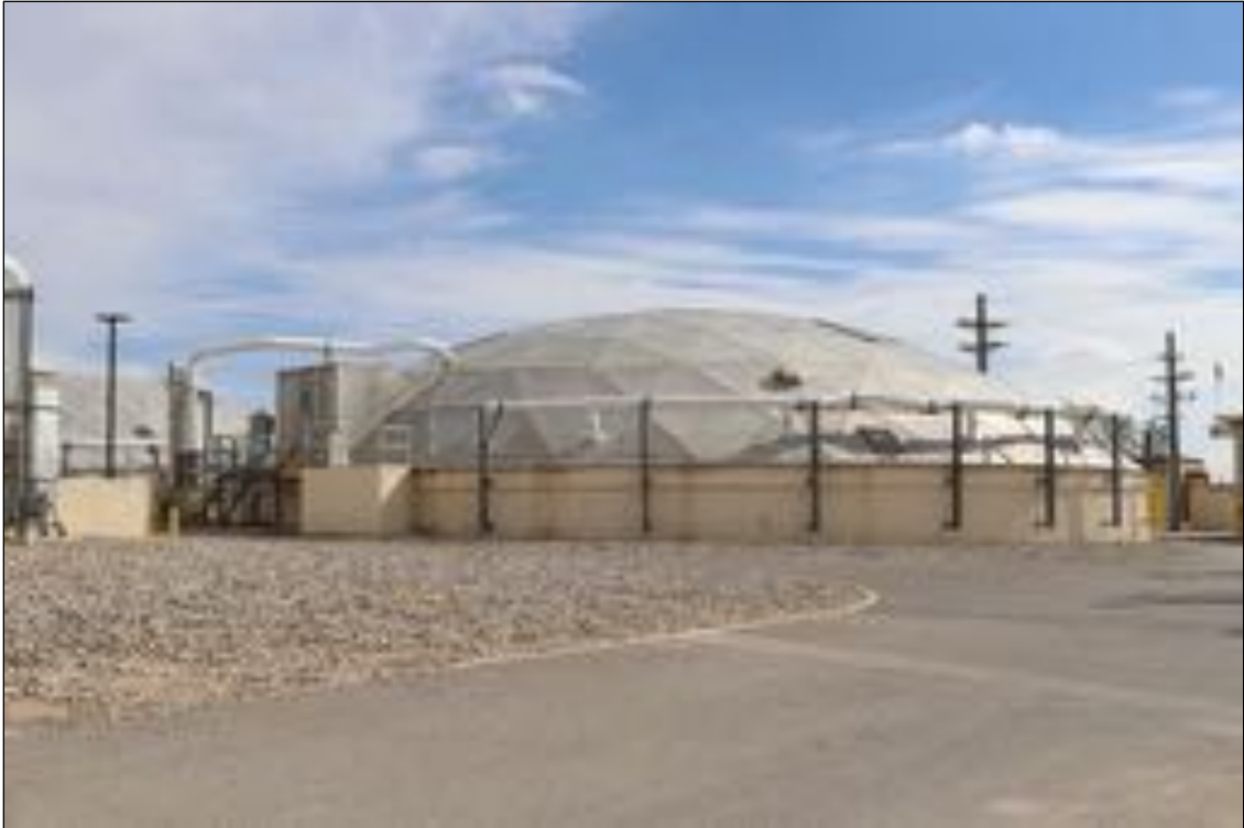
Figure 260. Digestion Tank, looking southeast.
