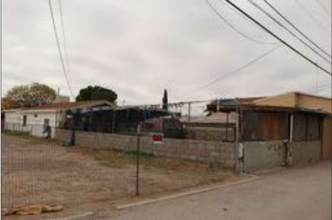
Figure 144. 3721 Findley Avenue (Residence) rear, looking southeast.
