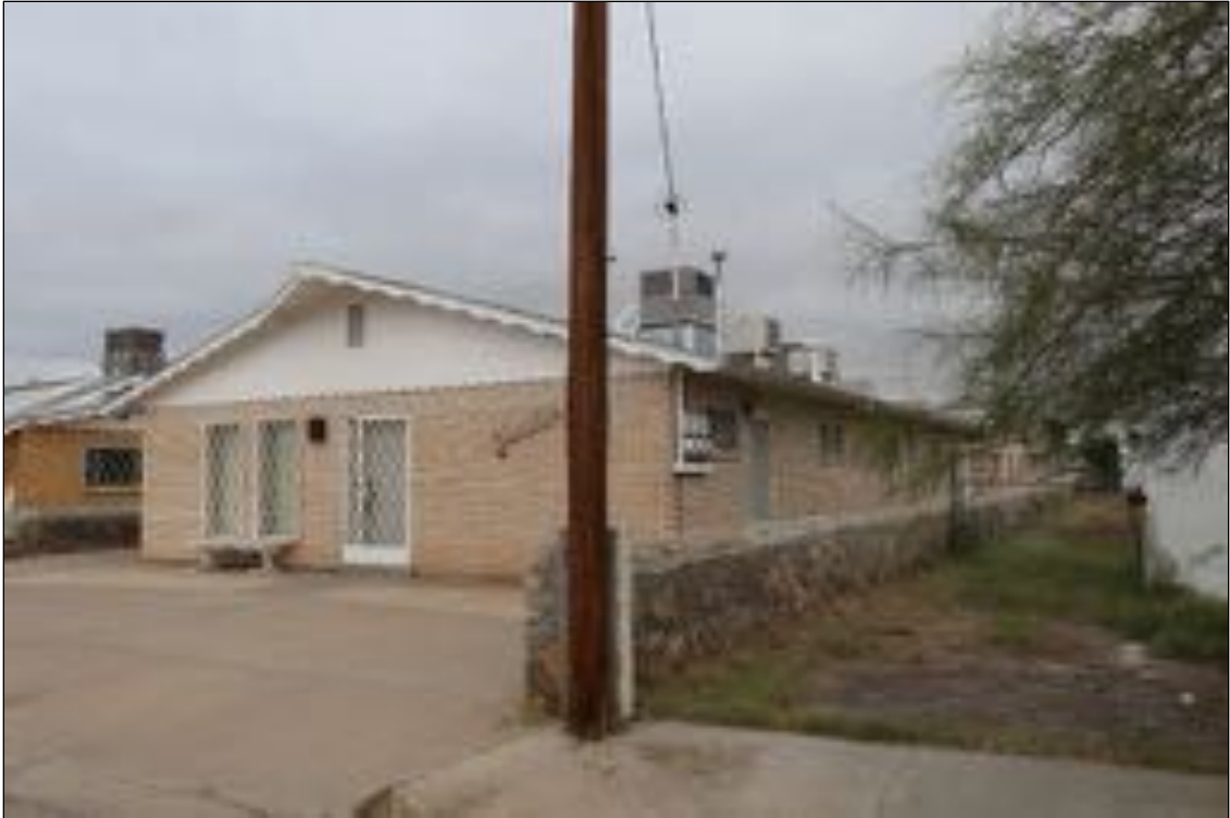
Figure 54. 4005 Oak Court (Residence), looking northwest.
