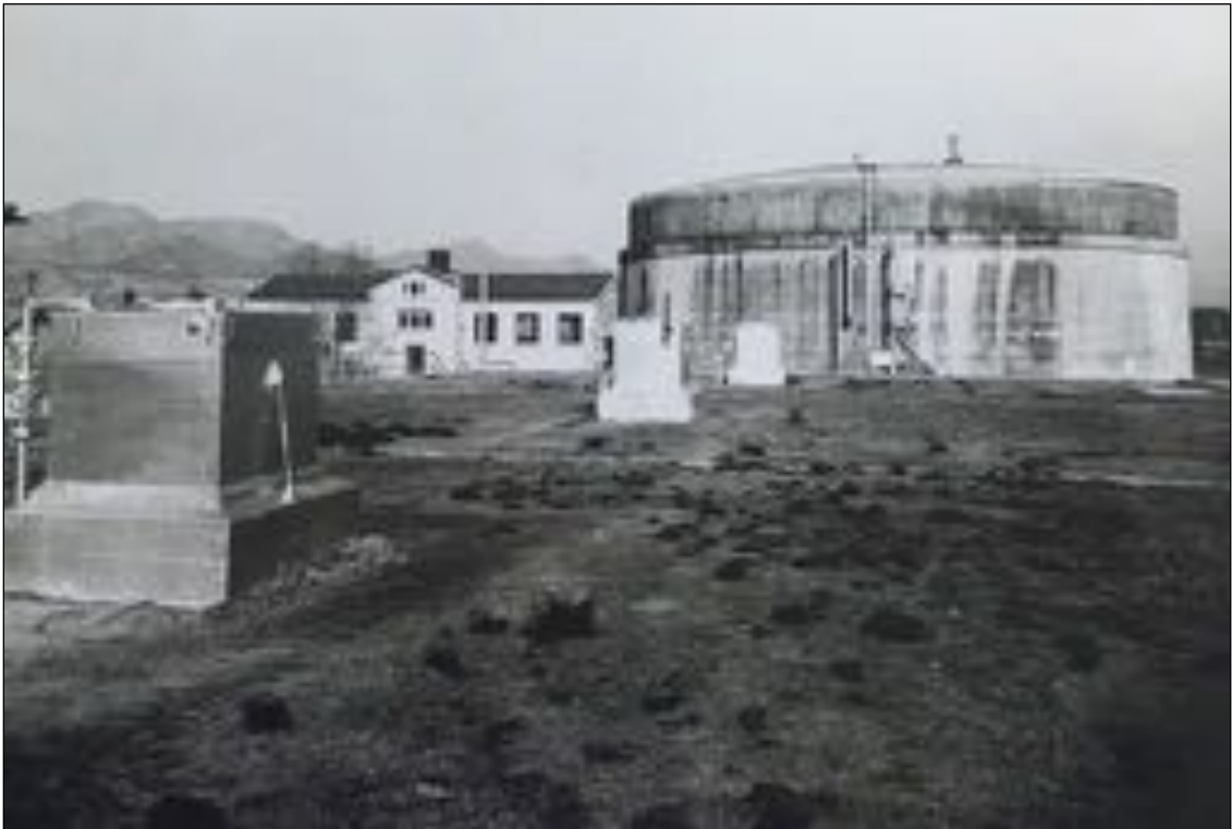
Figure 253. Shop, former Pump House, historic photograph ca. 1943, looking southwest.
