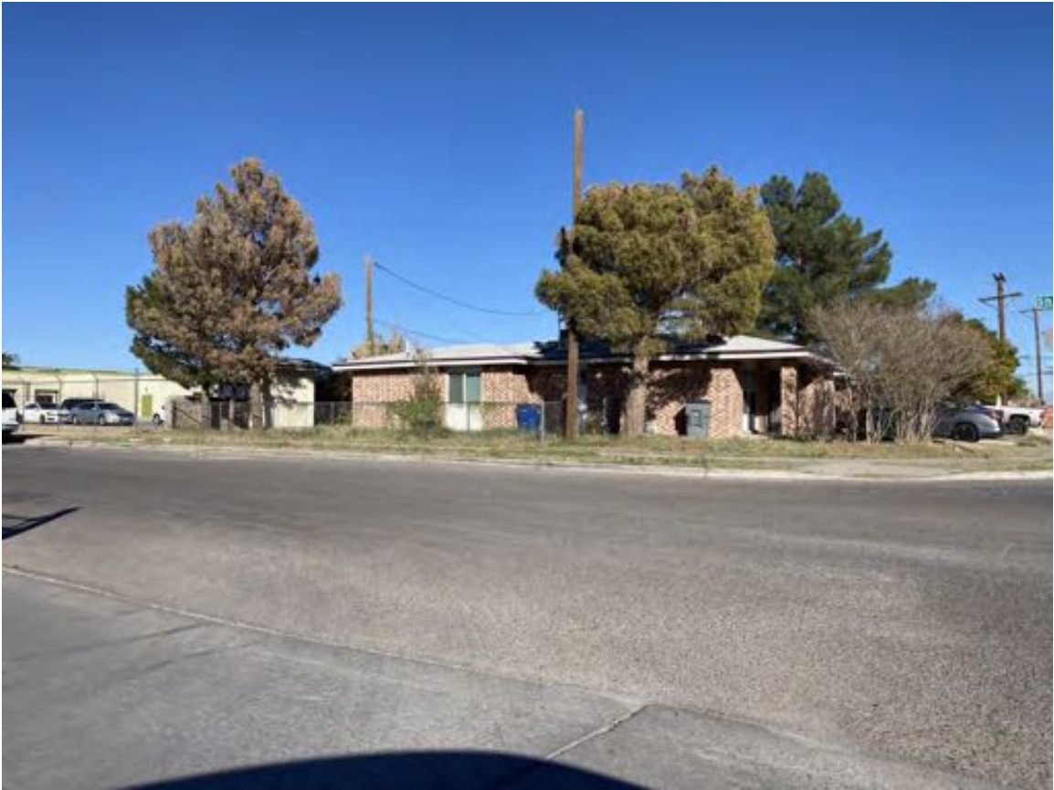
Photograph 18: View looking east across Shelter Place of the Salvation Army building and residences east of the County property.
