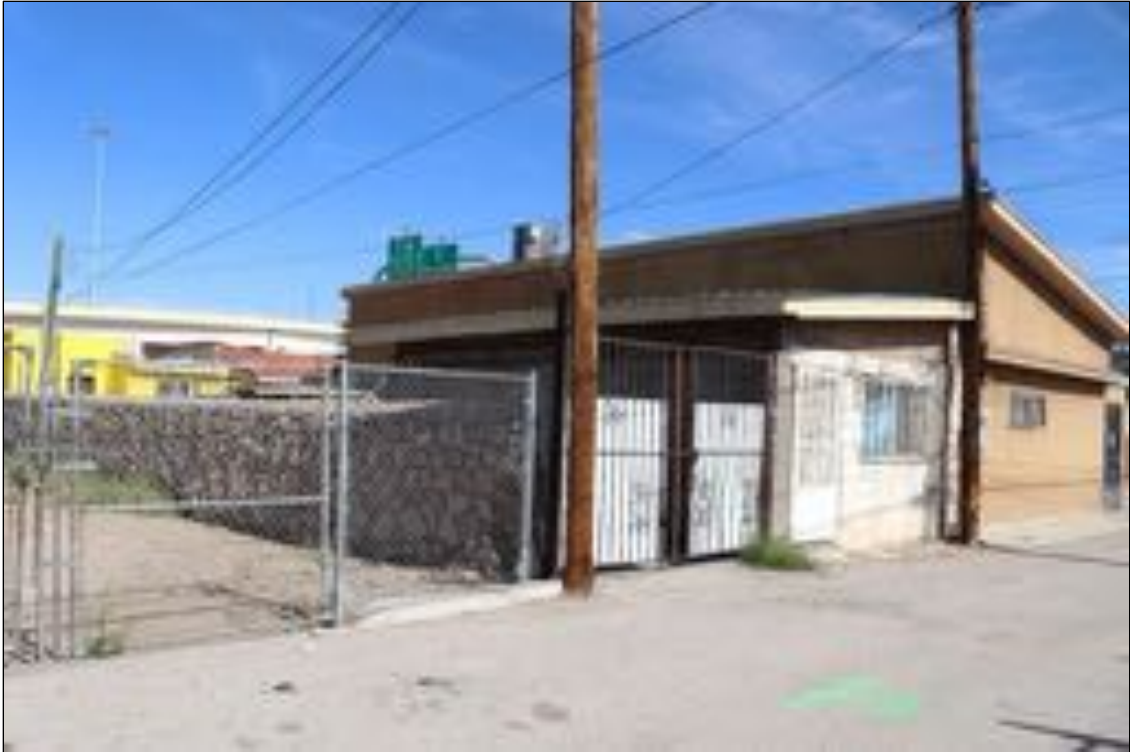
Figure 192. 3820 E San Antonio Avenue (Residence) rear, looking northeast.
