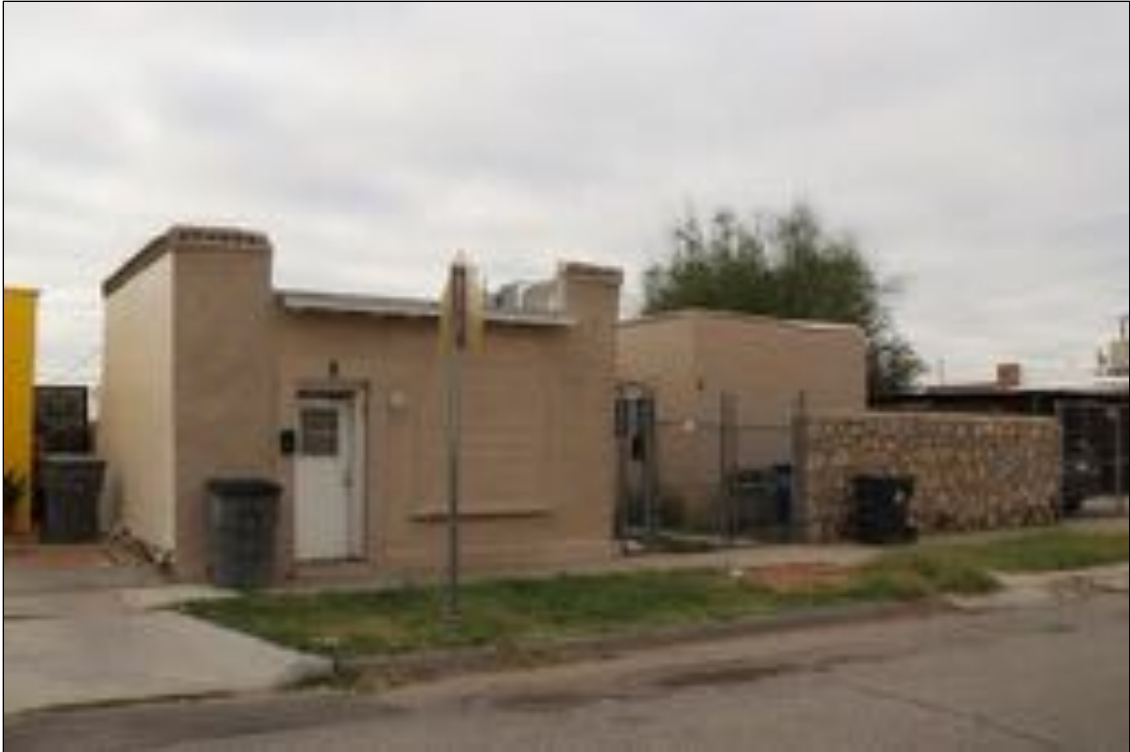
Figure 189. 3816 E San Antonio Avenue (Residence), looking south.
