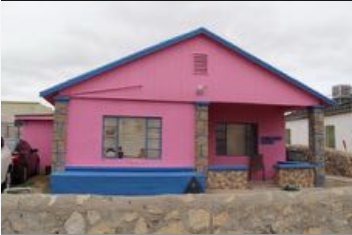
Figure 94. 211 Hardesty Place (Residence), looking west.
