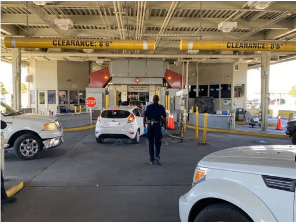
Photograph 4: View looking south towards the secondary vehicle inspection building.
