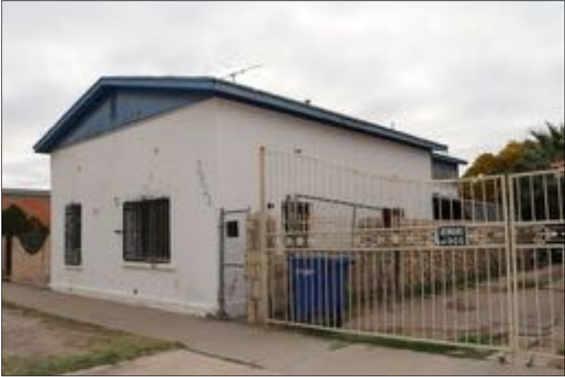
Figure 195. 3824 E San Antonio Avenue (Residence), looking southeast.
