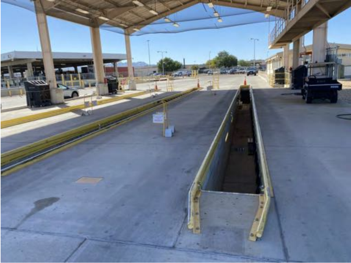
Photograph 9: View looking south of the truck inspection area.
