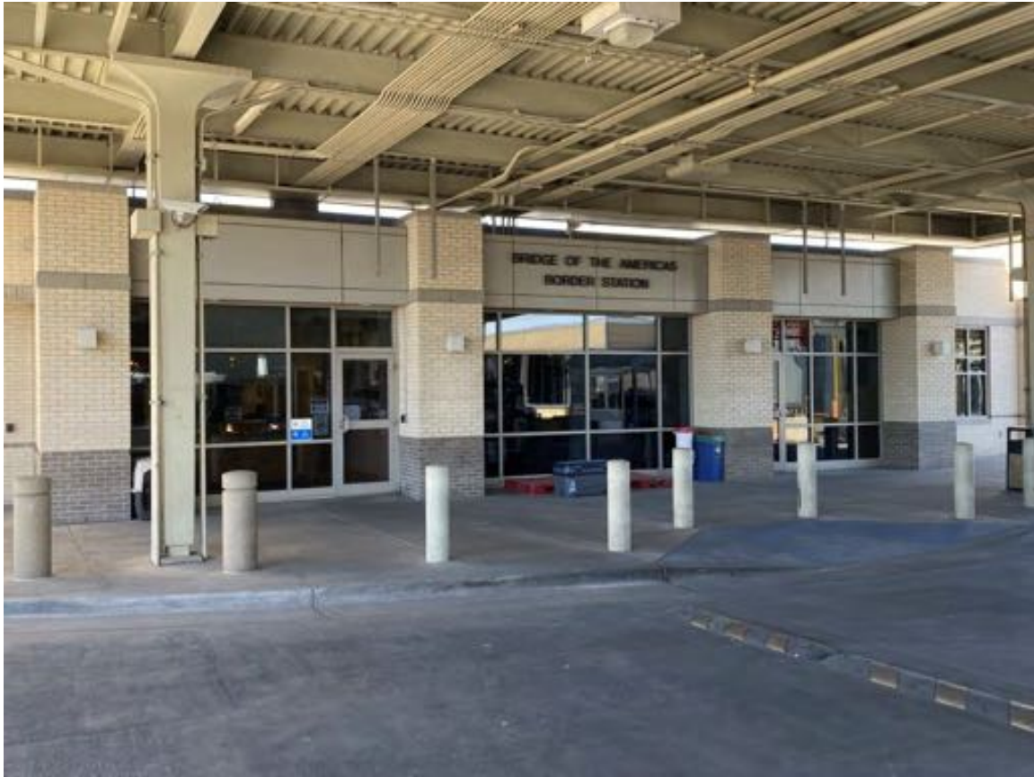
Photograph 5: View looking south of the secondary vehicle inspection building.
