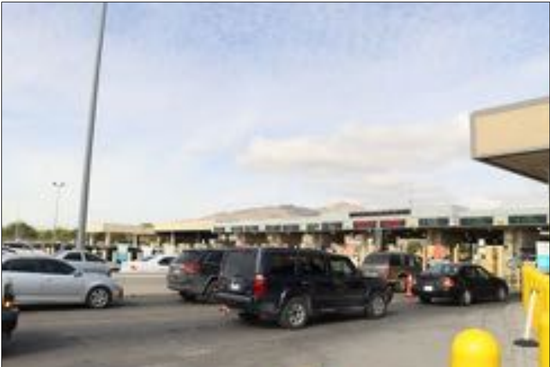
Figure 117. 3600 E Paisano Drive (Building K Primary/Secondary Inspection Canopy), south elevation of Primary Inspection Canopy (on the right), looking north.
