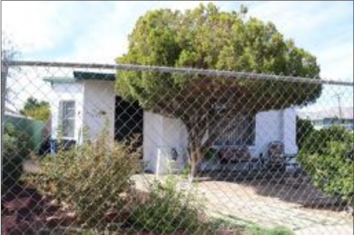
Figure 114. 407 Tobin Place (Residence), looking west.
