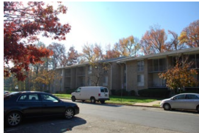
Franklin Park multi-family residential development
