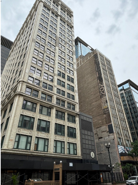
Figure 3.2-10. Picture Taken on South State Street showing East Elevation/Face of 220 South State Street
