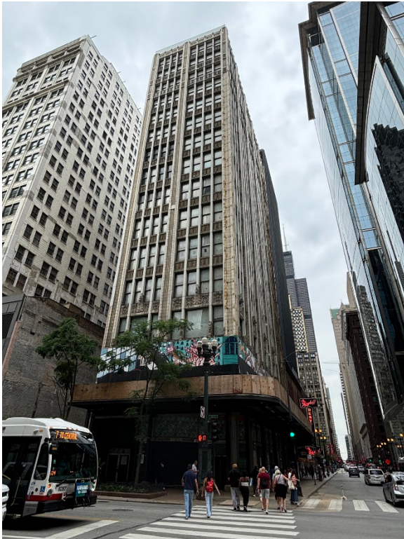
Figure 3.2-3. Picture Taken on South State Street showing East Elevation/Face of 202 South State Street
