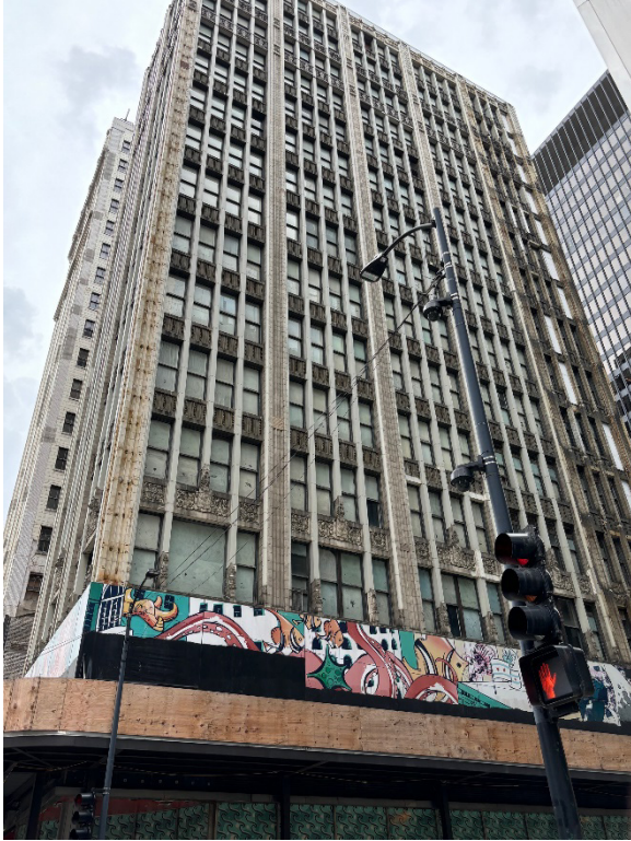
Figure 3.2-1. Picture Taken on Adams Street showing North Elevation/Face of 202 South State Street
