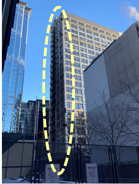
Figure 3.2-11. Picture Taken on Jackson Boulevard showing West Elevation/Face of 220 South State Street (circled)
