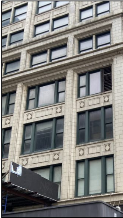
Figure 3.2-12. Picture Taken on South State Street showing South Elevation/Face highlighting Classical Revival Details of 220 South State Street
