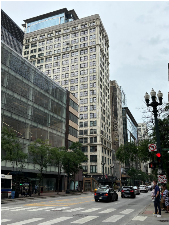
Figure 3.2-14. Southeast Corner of State Street and Jackson Boulevard looking North
