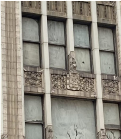
Figure 3.2-5. Picture Taken on South State Street showing East Elevation/Face highlighting Late Gothic Ornamental Detail of 202 South State Street
