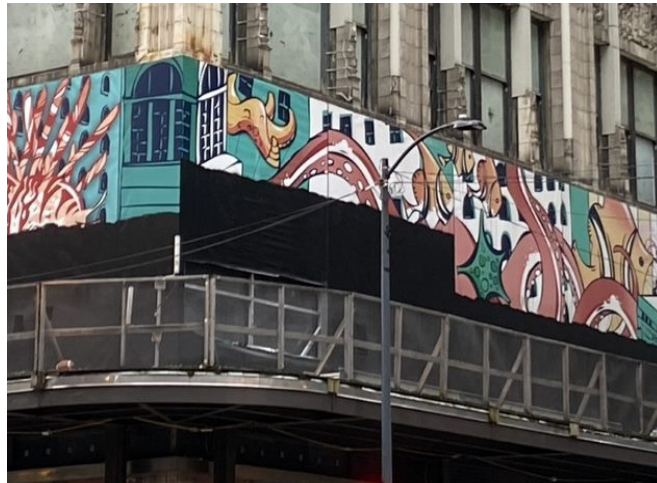
Figure 3.2-6. Picture Taken on Corner of South State Street and Adams Street showing North Elevation/Face highlighting Mural Detail of 202 South State Street
