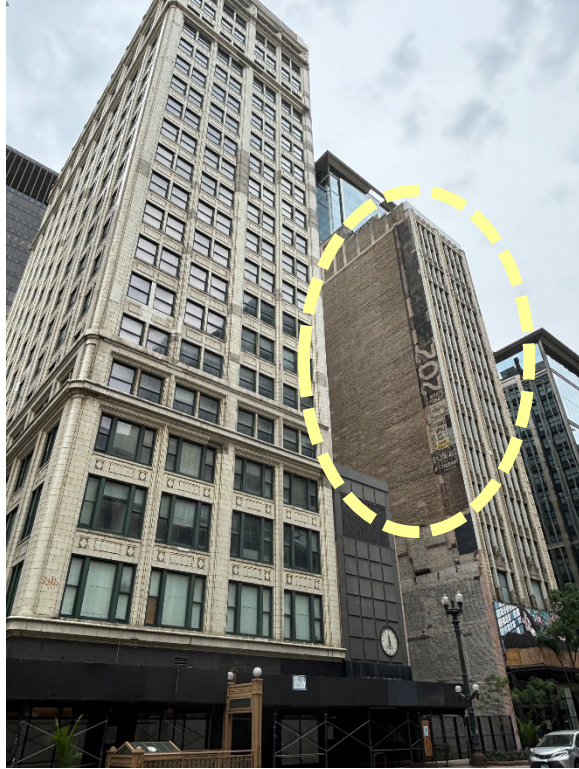
Figure 3.2-2. Picture Taken on South State Street showing South Elevation/Face of 202 South State Street (circled)
