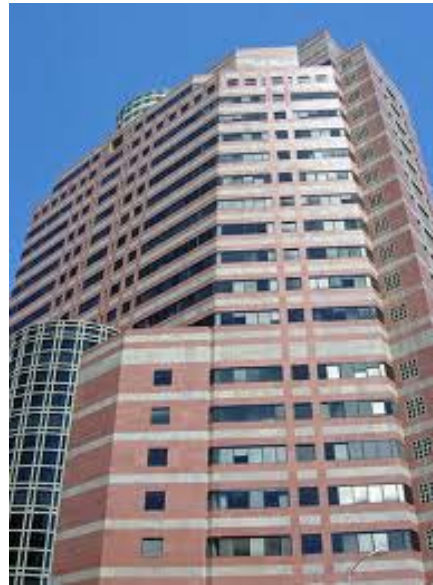
Figure 74. Roybal Federal Building
