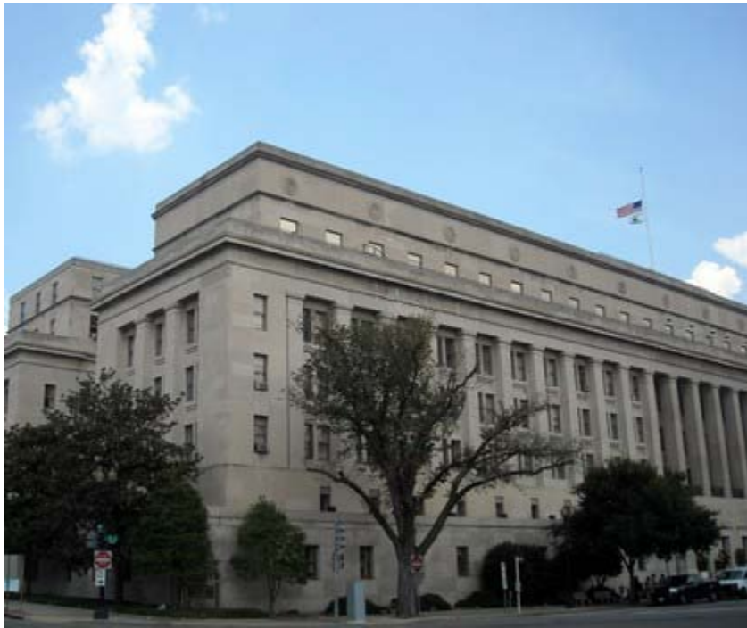
Figure 108: US Department of the Interior
