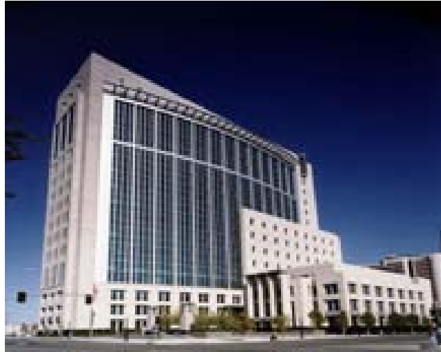
Figure 63: Robert Matsui Federal Courthouse, Sacramento, CA
