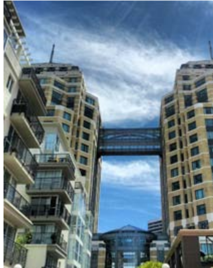
Figure 71: Ronald V. Dellums Federal Building at Oakland City Center
