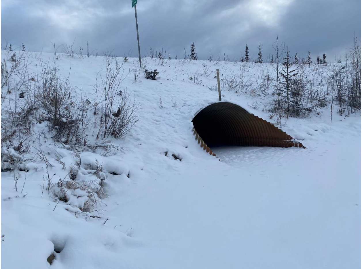
Figure 5. Bridge No. 7084 (culvert) at Desper Creek downstream opening
