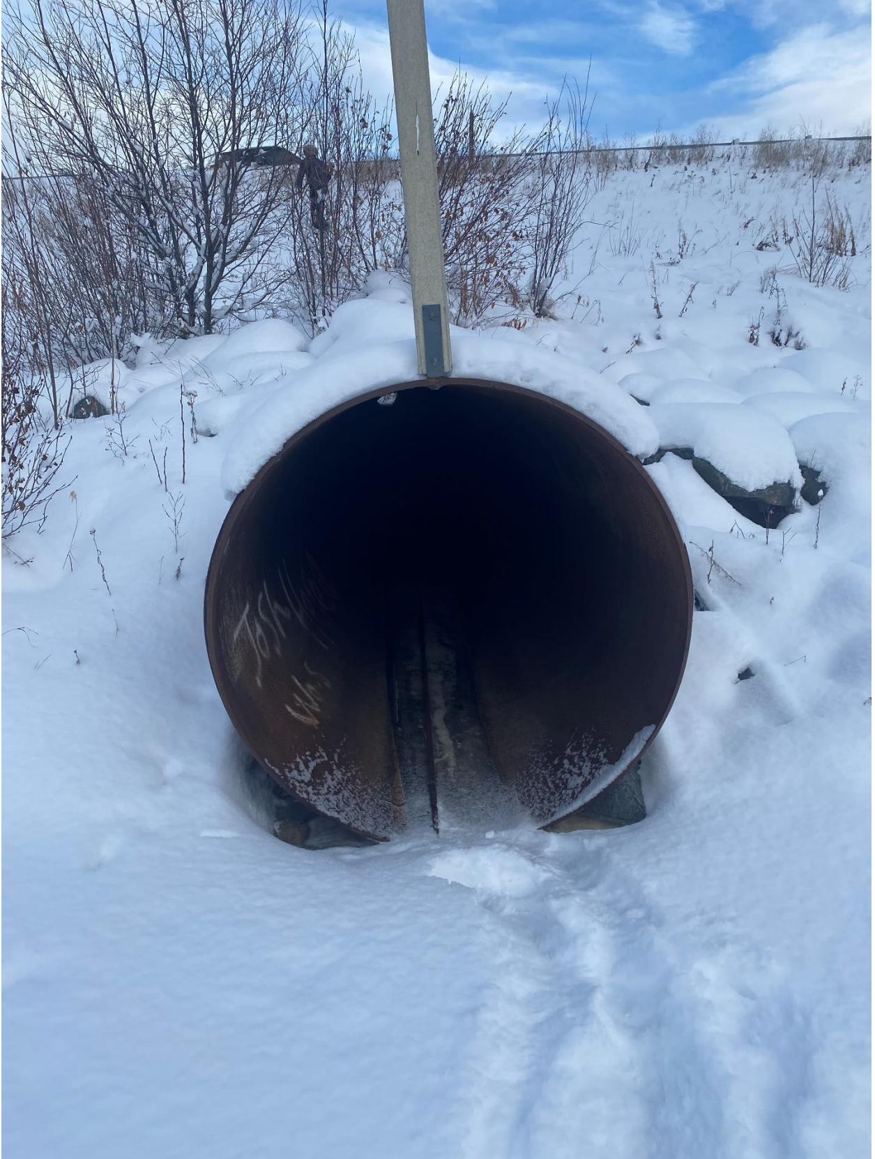
Figure 3. Steel pipe culvert near Alcan Land Port of Entry
