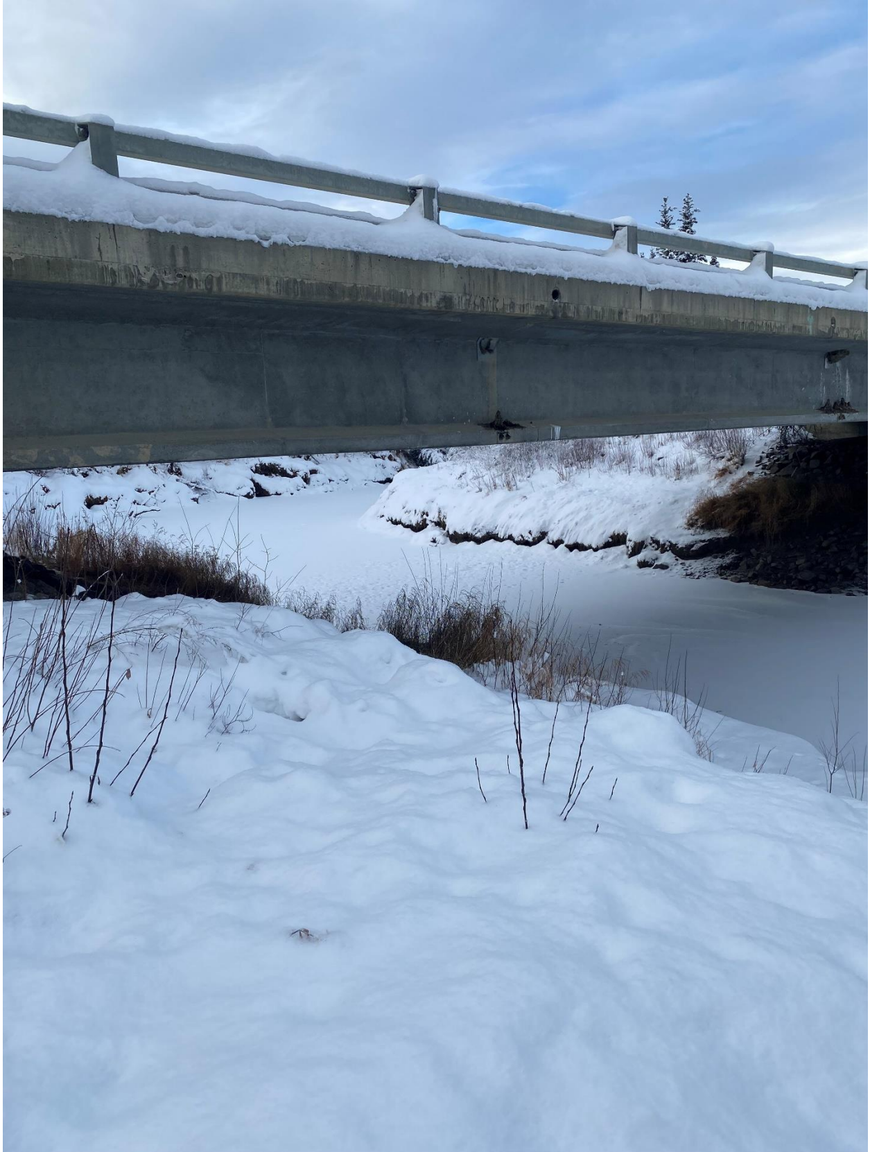
Figure 4. Bridge No. 0501 at Scottie Creek looking downstream
