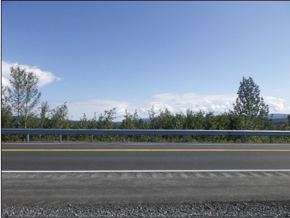
Figure 8. Overview from SPT016, view East (NLURA photograph).
