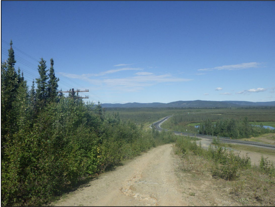
Figure 9. The Alaska Military Highway Telephone and Telegraph Line (NAB-00373) (NLURA photograph).
