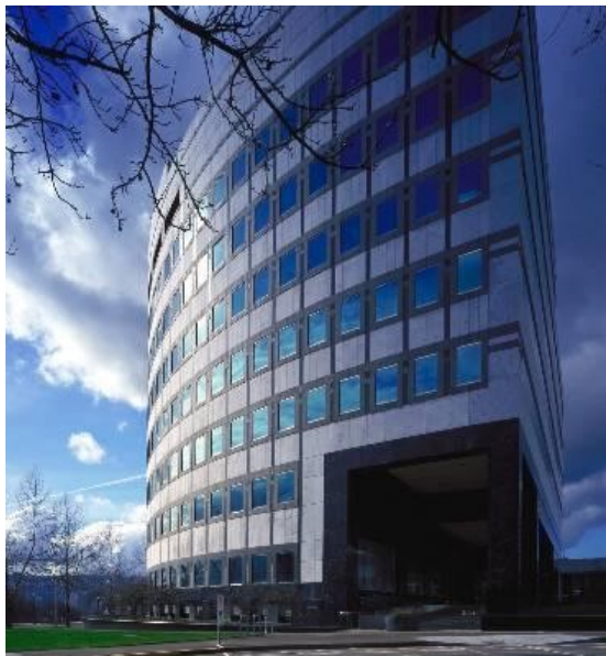
Bonneville Power Administration (BPA) Building, Portland, Oregon
