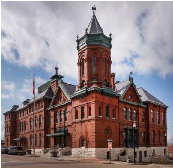
U.S. Post Office and Custom House, Vicksburg, Mississippi Highsmith, Carol M., 1946, photographer
