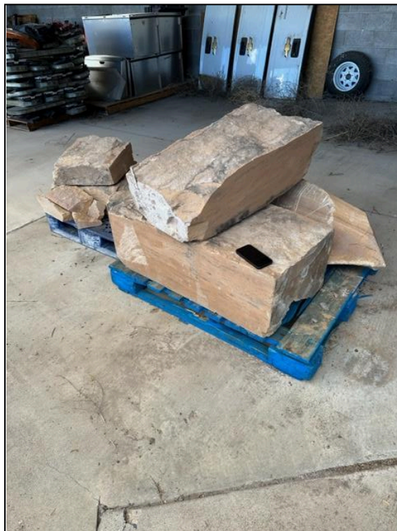
Figure 15. Kit Carson monument, damage to the obelisk (photo taken September 2023).
