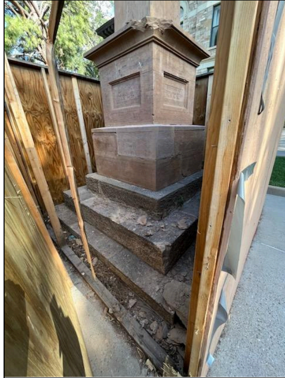
Figure 14. Kit Carson monument, damage to the monument. Note fragmented remains (photo taken September 2023).
