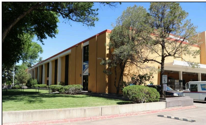
Figure 6. Joseph M. Montoya Federal Building and Post Office, looking northwest (photo taken June 2024).
