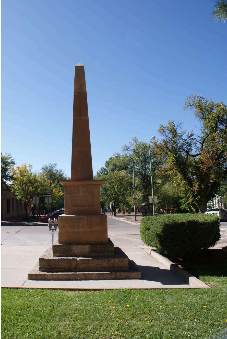
Figure 10. 2019 condition of Kit Carson monument.
