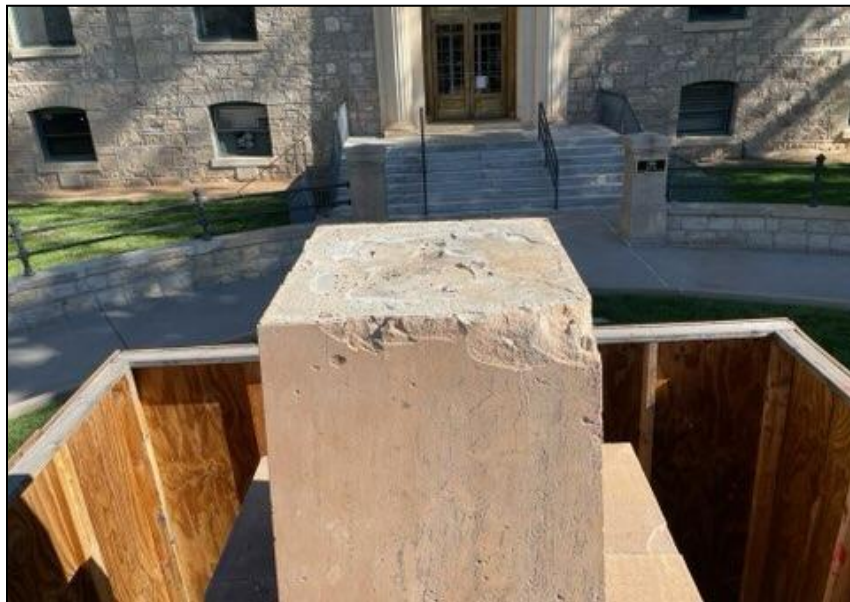
Figure 13. Kit Carson monument, damage to the obelisk (photo taken September 2023).
