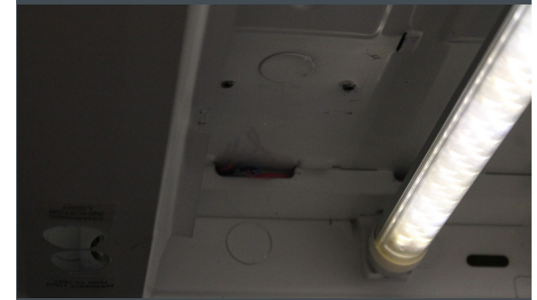
Low-quality TLEDs can have a “pixelated” appearance. Photo credit Michael Myer, PNNL
