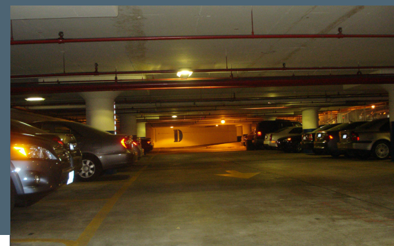
Integral occupancy sensor in parking garage luminaire increases output when motion is detected. Photo credit Akoya, U.S. DOE
