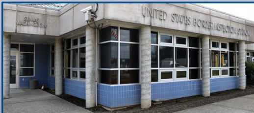
SUMAS LAND PORT OF ENTRY PHOTO CREDIT: GSA
