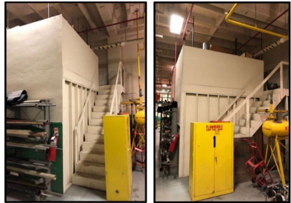
Photographs M1 and M2 Temporary mezzanines
