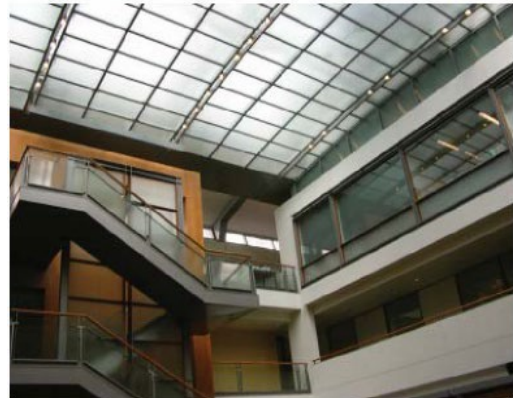
Example of a skylight above an enclosed courtyard.
