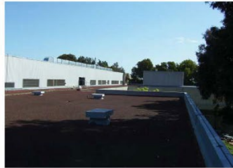
Example of a building that has no attic space. This is a roof with a mechanical penthouse.
