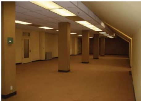
Example of attic space.
