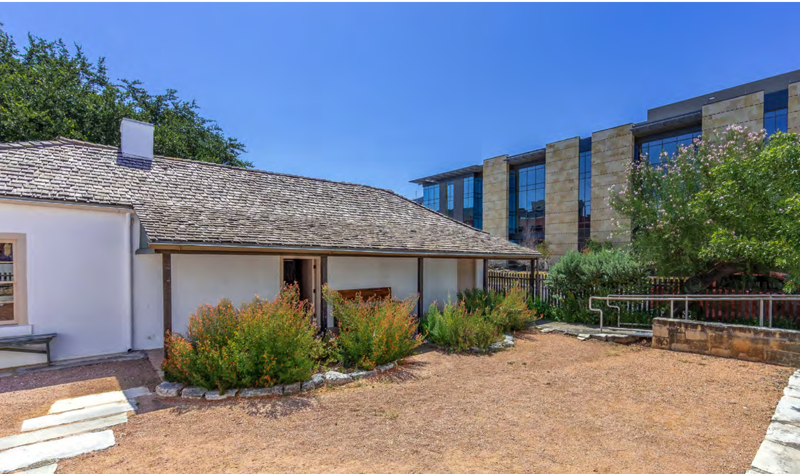
The courthouse's north elevation, seen from the grounds of Casa Navarro
